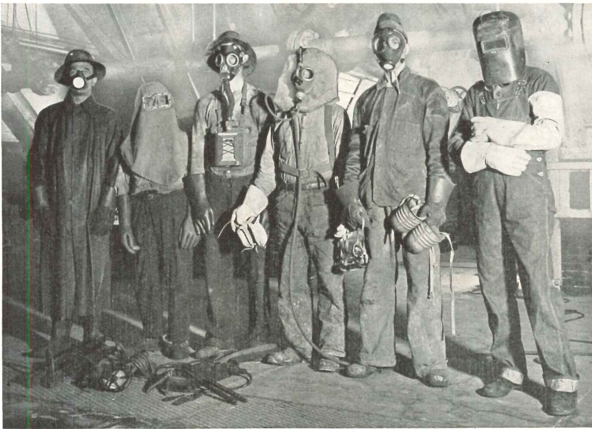
Different types of safety clothing designed for different kinds of atmosphere.
