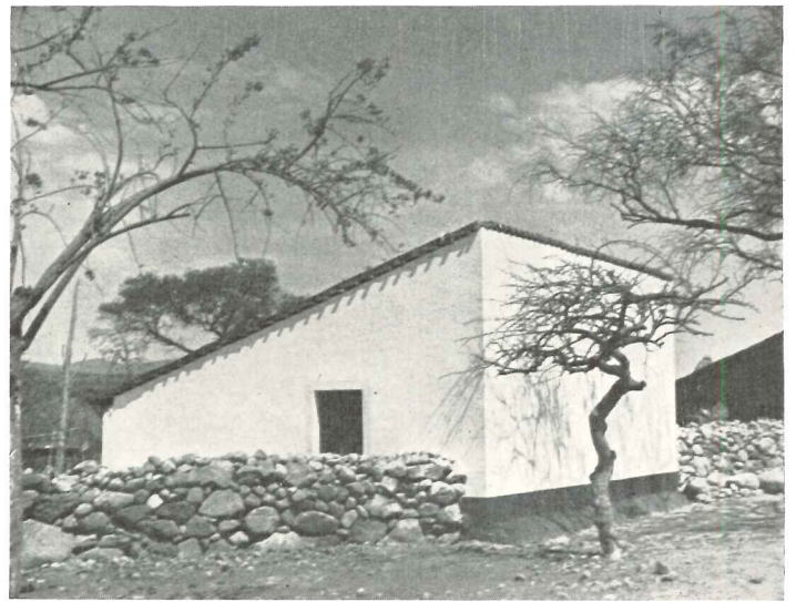
ADOBE WALLS, PLASTERED — TRADITIONAL METHOD
