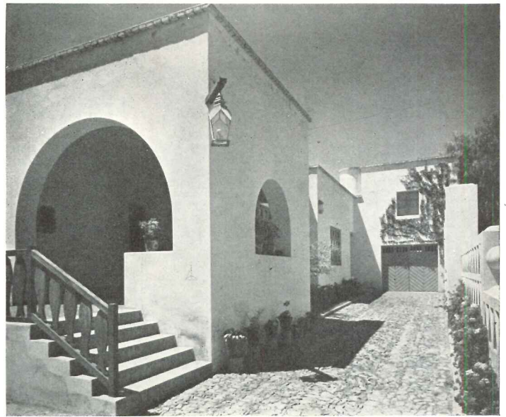
ENTRANCE AND GARAGE
