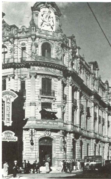
END OF 19TH AND BEGINNING OF 20TH CENTURY THE BANK OF LONDON AND MEXICO
