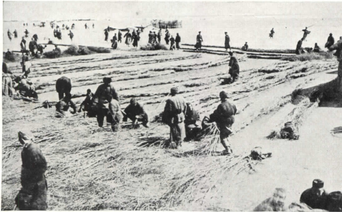
MORE THAN 5,000 TONS OF HEMP and tens of thousands of willow branches were used in making fascines to build a 600-mile dike. The branches are laid out in straight rows 50 feet long along the ground, twisted together and then tied with hemp rope.
