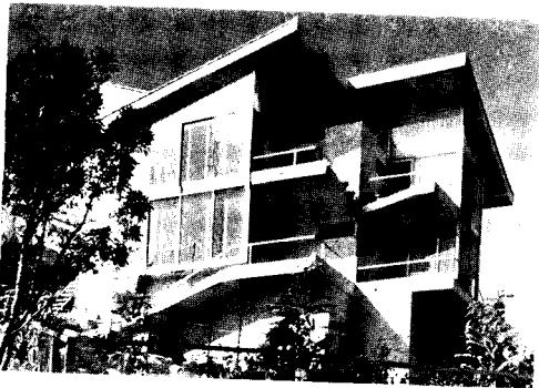
W. P. Woodcock Van Patten House, Los Angeles, R. M. Schindler, architect
