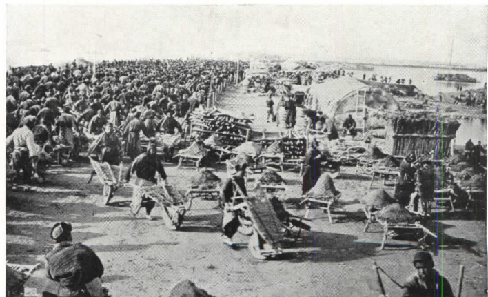
WHEELBARROWS WOVEN FROM WILLOW BRANCHES and manned by coolies, carried supplies to danger points on levees. Wheels and framework are hand hewn, and fastened with hemp rope.
