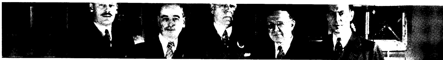
Five men standing on Herculite tempered plate glass specially processed by heat and chilling, demonstrating the resistance to an impact seven to eight times greater than ordinary plate glass.
