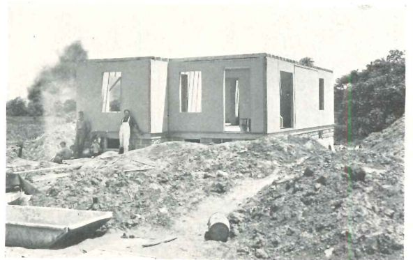
And 4 hours labor sees all partitions up, job ready for roof framing with precut rafters.
