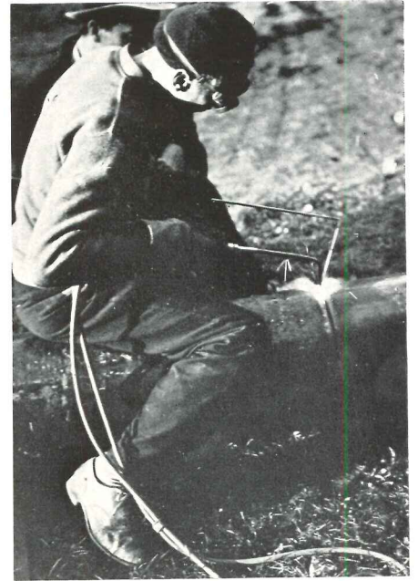
3. WORK OF EACH WELDER IS TESTED BEFORE HIS EMPLOYMENT IS PERMITTED. COUPONS, 2" x 10", ARE CUT FROM TRIAL WELDS ON SMALLEST DIAMETER PIPE TO BE USED. THESE ARE FIELD-TESTED BY BEING BENT AT INSIDE OF WELD THROUGH 180°. NO FRACTURE SHOULD OCCUR WITHIN THE WELD. NO UNEVENNESS IN EVIDENCE. NO PROJECTION OF METAL INTO INSIDE OF PIPE. LABORATORY TEST FOR HYDROSTATIC AND TENSILE STRENGTH.
