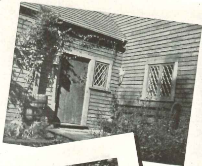
Architect, Jerome B. Foster, Winchester, Mass.
