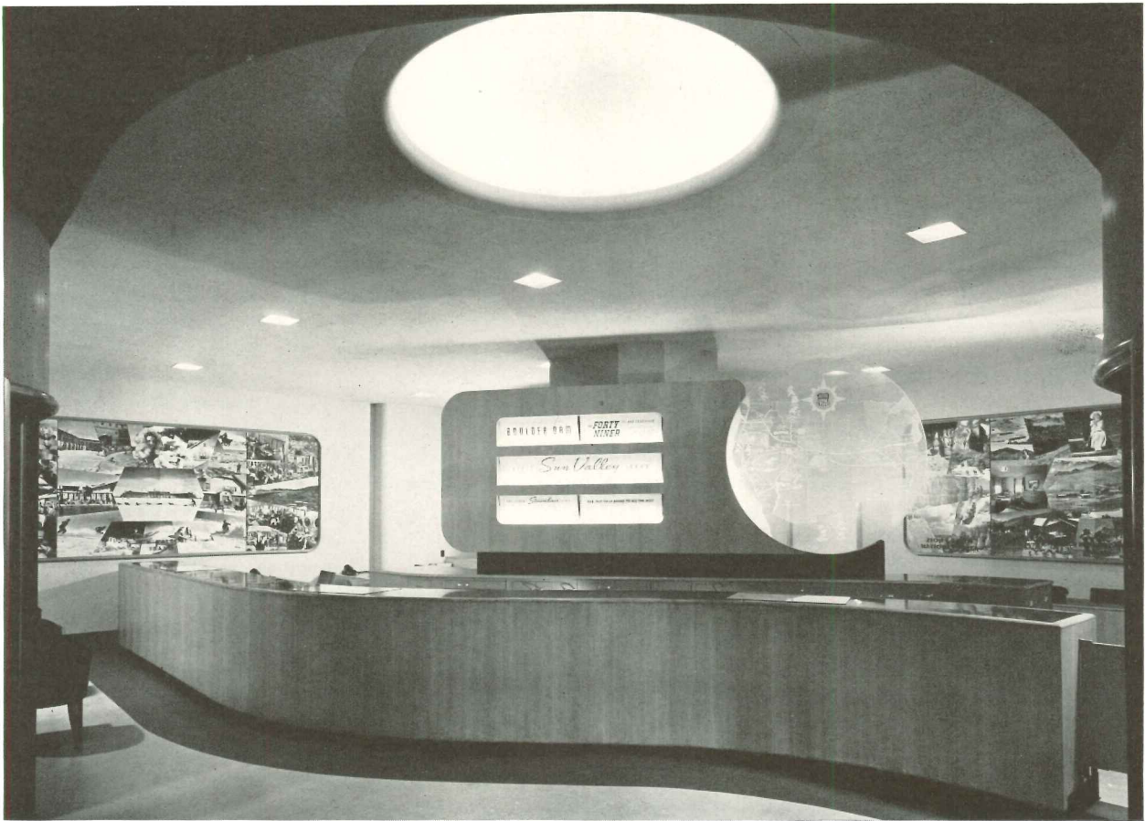
View of public counter. Front face of counter and frame behind it are oak, of natural finish and lacquered.
