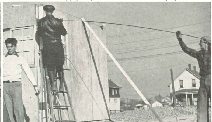
6. Panels are tied together with steel rods and bolted at corners; walls are drawn into rigid units. . . .
