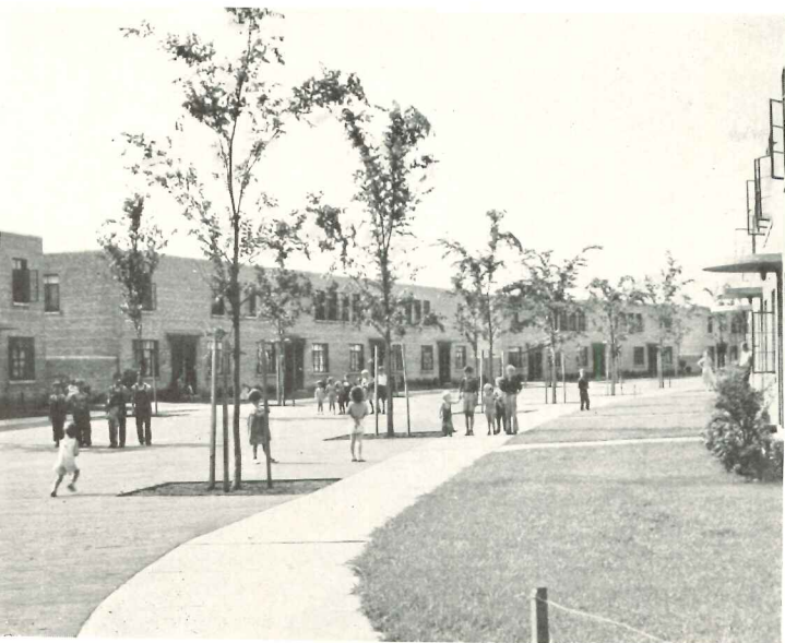
Play area surfacing, Trumbull Park Housing, Chicago
