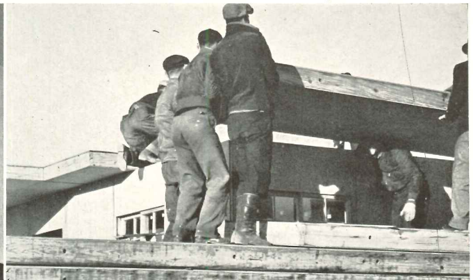
8. When the walls have been completely assembled and bolted together, the roof panels are placed in position.
