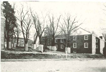
Grand View Heights Apartment Project, Lancaster, Pa. Architects: A. R. Clas Associates, Washington, D. C., Floyd A. Kline, Lancaster, Pa. Gen. Contractors: C. H. Shufflebottom, Lancaster, Pa.
