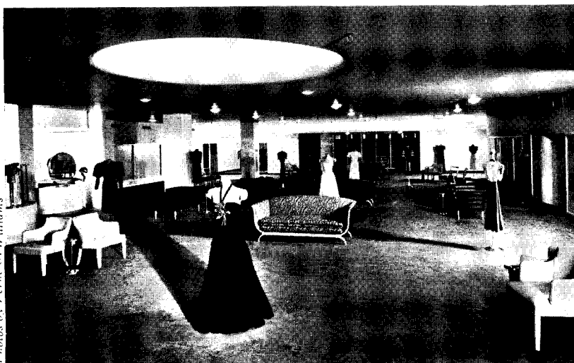
Women's dress department, third floor. Flush-type lighting fixtures are supplemented by indirect trough neon illumination.
