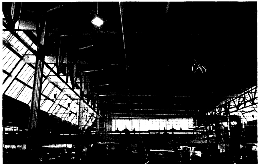
Main assembly line, showing some of the fifteen hundred 450-w. mercury lamps.
