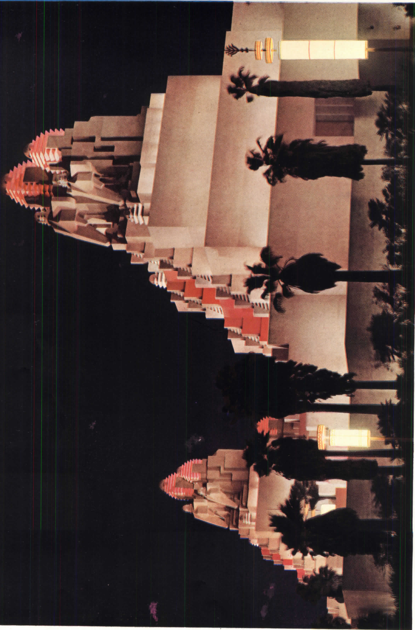
PLATE 5. Highest intensities and lightest colors have been widely used on those elements primarily designed to be seen from afar. Thus the brilliantly lit West Facade, with its monumental entrances, actually serves as a huge sign which dominates the city's eastern horizon and intersects its traffic lanes to the mainland. Colors are concentrated at the entrances.
