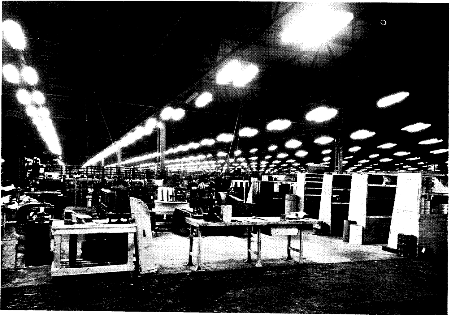
Above, 100-w. Cooper-Hewitt fluorescent lamps installed in pairs. Below, underfloor power duct; all risers run up columns. System provides maximum flexibility and frees overhead space of wires, etc.
