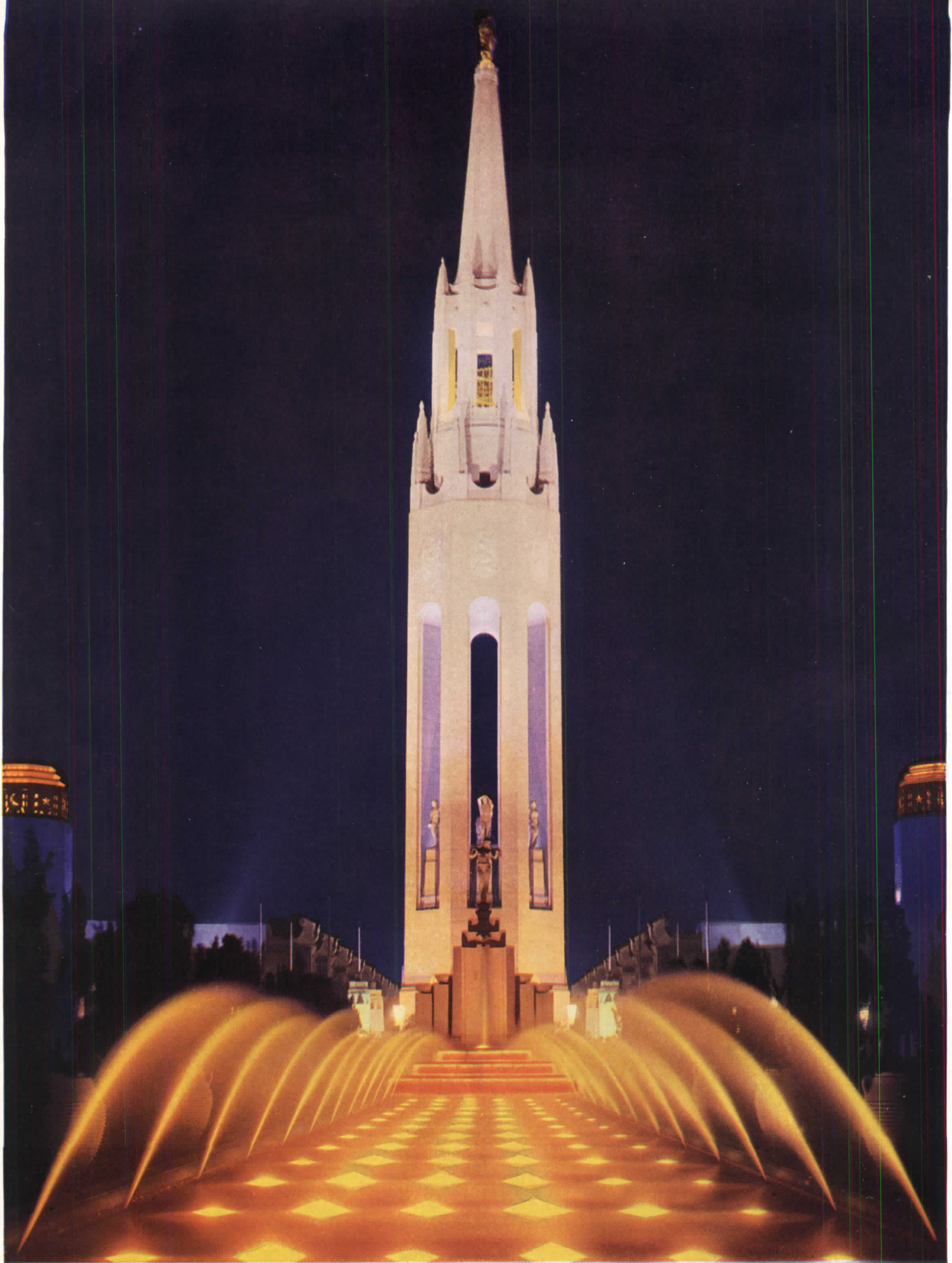
PLATE 11. Beginning with a warm amber at the base, the Tower of the Sun changes gradually to a white of increasing intensity at the top. Relief lighting is blue at the base, straw yellow at the belfry, amber at the pinnacle (Figs. 18, 19 and 20). The surrounding Court of Honor is mainly illuminated by this reflected light, although 24 decorative street lighting units supplement the design.
