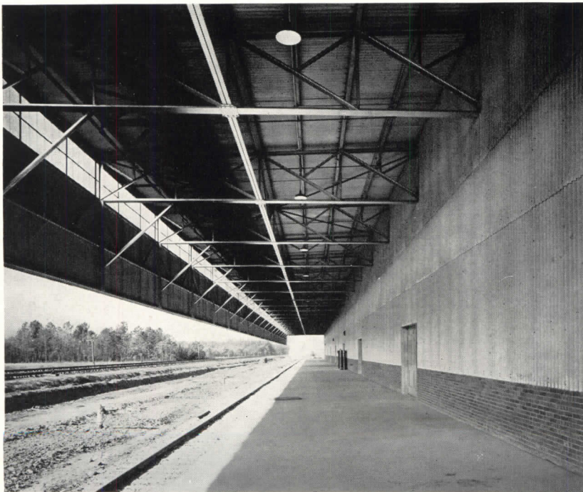
Shipping-platform width permits carload lots to be assembled without obstructing passage of trucks or human beings.
