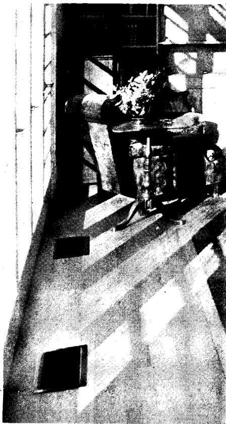
5. Floor outlets near an exposed wall counteract the cold air which sweeps down the outer wall and across the floor.
