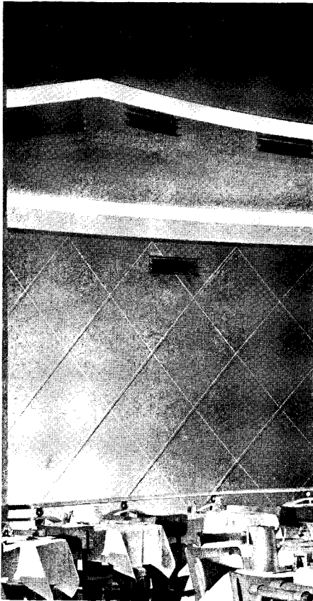
2. Grilles of supply ducts were designed for minimum obstruction to air flow and maximum directional control.
