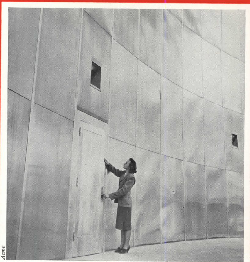
Air Conditioning Mt. Palomar observatory. Between inner and outer aluminum-plate walls is a 4-ft. plenum chamber.
