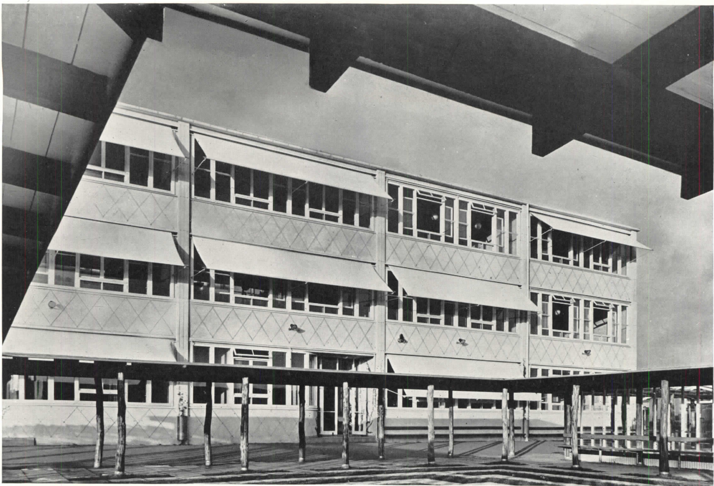
Main building: Load-bearing partitions facilitate use of continuous fenestration. Exterior walls are covered with colored stucco.
