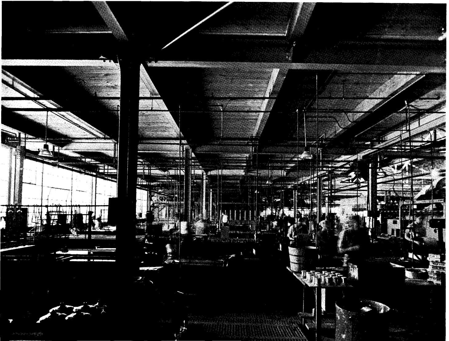
Plating Department: Acid-bath fumes caused wood roof deck to be used; on steel framing only is periodic painting needed.
