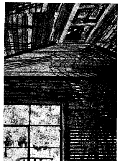
Panel-heating installation; copper tubing mounted on face of laths.
