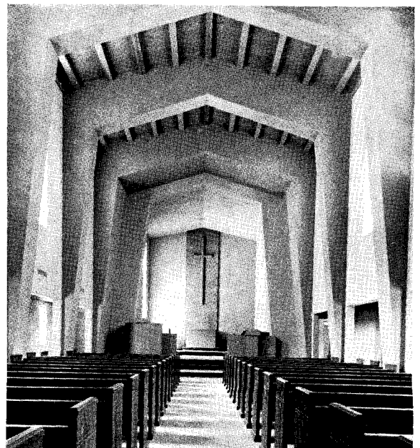
Structural form is the dominant motif of the interior.
