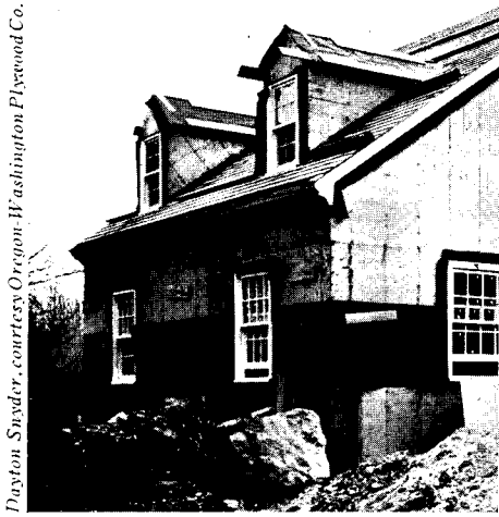
Complete stoppage of air infiltration is necessary; it may be achieved, as here, by using plywood sheathing plus attention to detail at openings.
