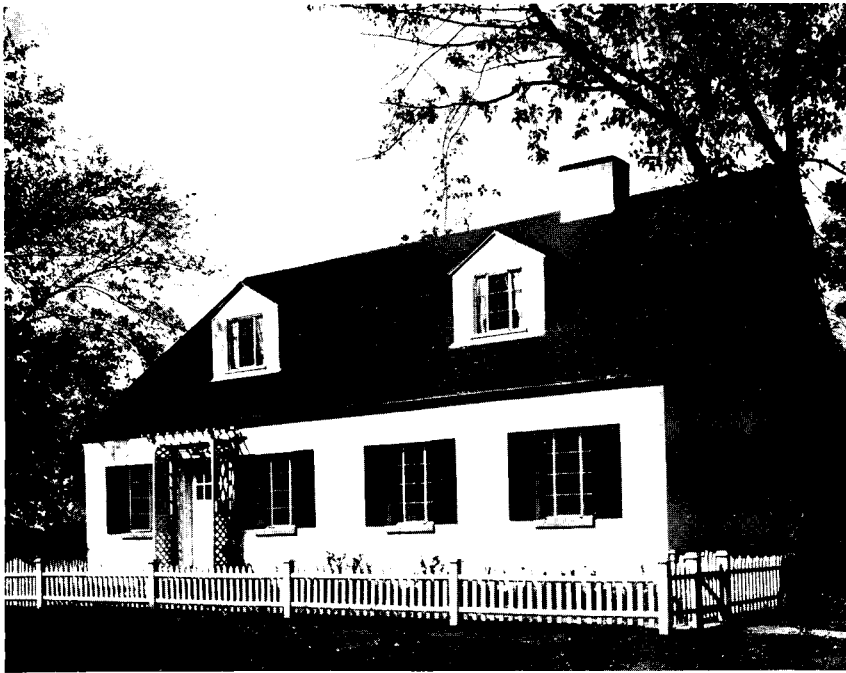
House in Troy, Wisc., built with patented molds distributed by Hollow Concrete Wall Mold Co.; at right, construction method. Mix is relatively dry, well tamped; top of each pour is left rough for bonding. Forms may be
