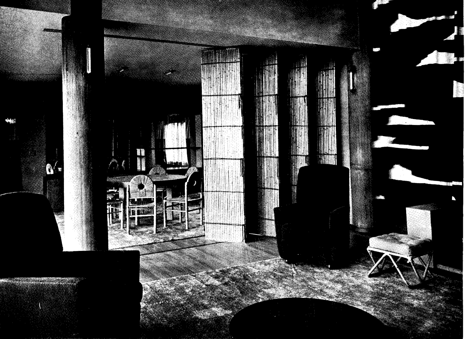
Wood structure system devised by Antonin Raymond, architect: essentially post-and-lintel construction with curtain walls.
