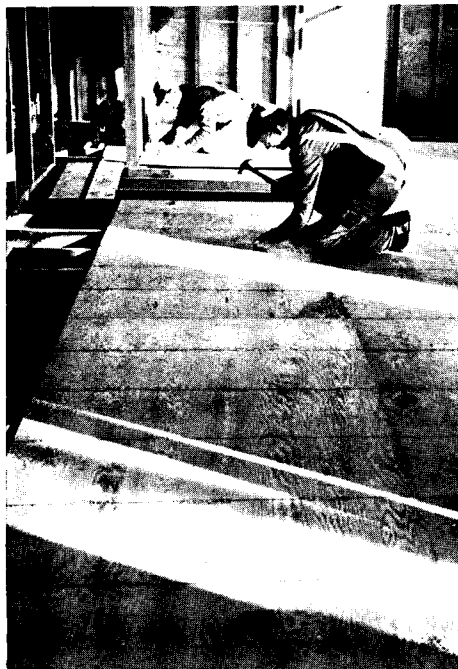
R. B. Edward house: laying subflooring of five-ply, 4 by 8 ft., 5/8 in. thick, unsanded "Plyscord."
