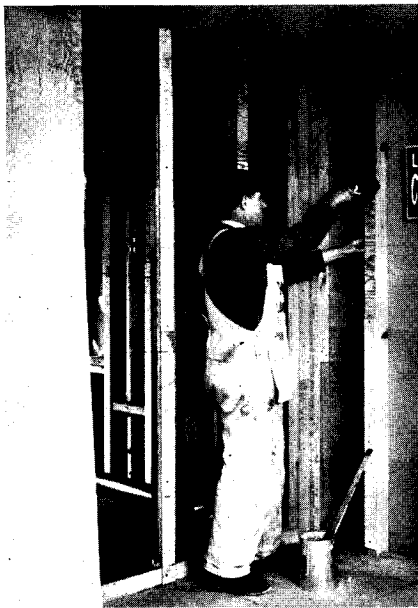
Installing plywood so as to minimize shrinkage effects. (See pages 90 and 96)
