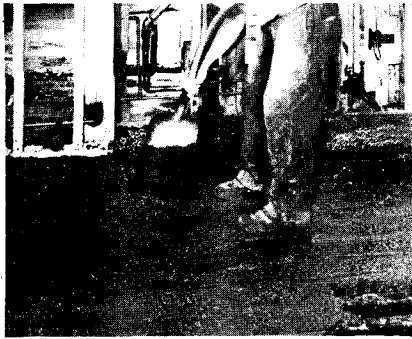
Pouring cement grout fill on cellular steel floor framing, providing incombustible floor structure.
