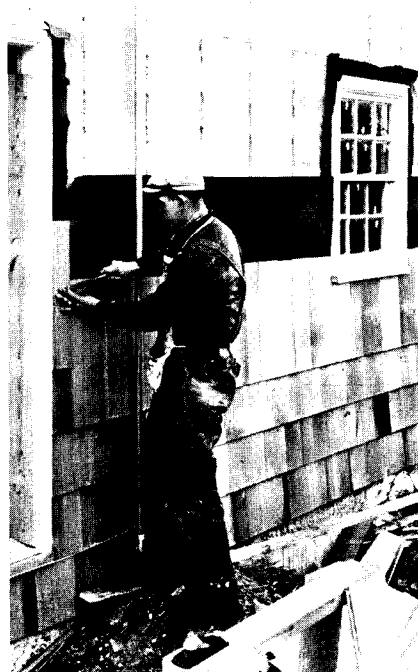
Shingling the Edward house. Use of plywood and prevention of wind-leakage at openings reduced air-infiltration so greatly that use of wall insulation was considered uneconomical. However, roof insulation was included. Specifications were prepared in cooperation with the Oregon-Washington Plywood Co., using the "Uniwall" system.
