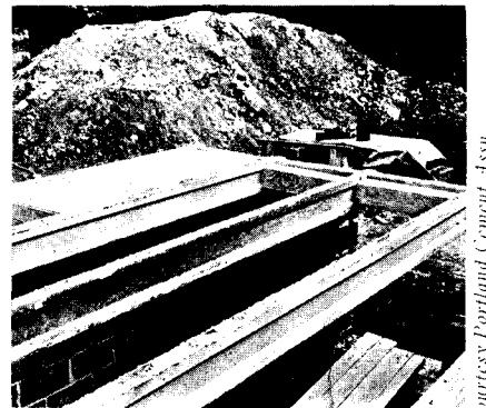
Precast concrete beams and field-cast floor slab
