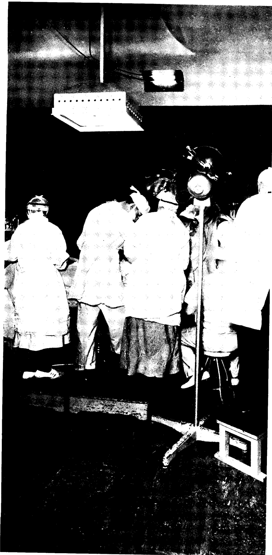
Direct ultraviolet irradiation in the operating room of a hospital in Boston protects the surgical incision against infection by air-borne bacteria.
