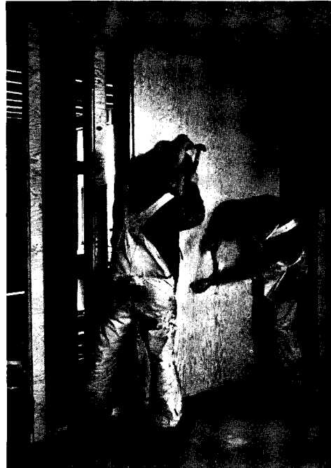
Applying interior plywood: in "Uniwall" system used, 1/4-in. plywood is both glued on and nailed with finishing nails.
