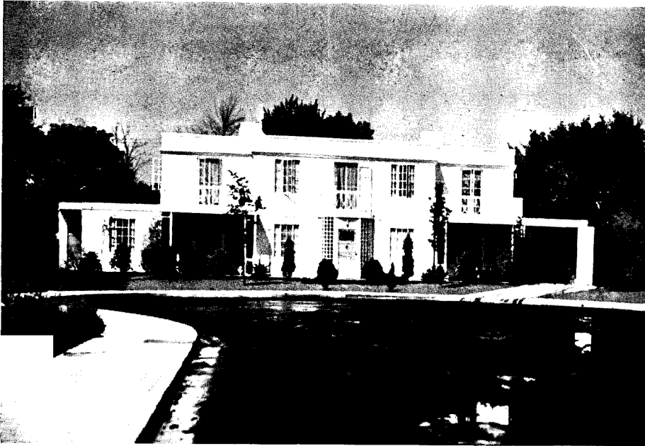
Hobart all-welded steel houses are completely shop-fabricated, trucked to the site, placed on the foundation, and hooked up to utilities. Walls and floors are thin, double-faced, reinforced steel, welded together and packed with insulation. Center, below, forming a door panel; and, bottom, houses on the production line.
