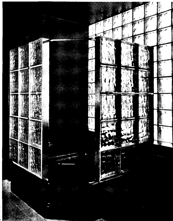
Glass-block partitions are used in the bathroom. Above is the corner tub, with side walls of glass block set in a metal frame, and a curtain bar provided over the opening.
