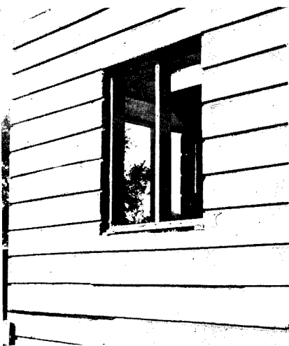
Weakened plane joints accommodate concrete shrinkage.
