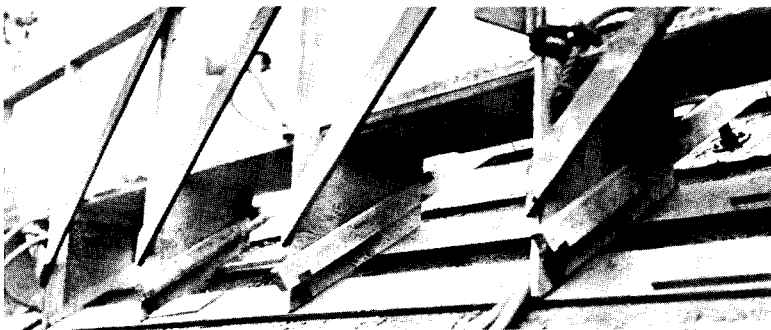
"Sky-hook" vacuum-concrete forms: 1, laboratory demonstration showing, at bottom, pour from which form has just been removed; above that, form held in place by atmospheric pressure; top, form supported on second-course form. 2, gable-end of a house in Westchester County, N. Y. 3, roof of same house. 4, scaffolding supported on unset, dehydrated concrete
