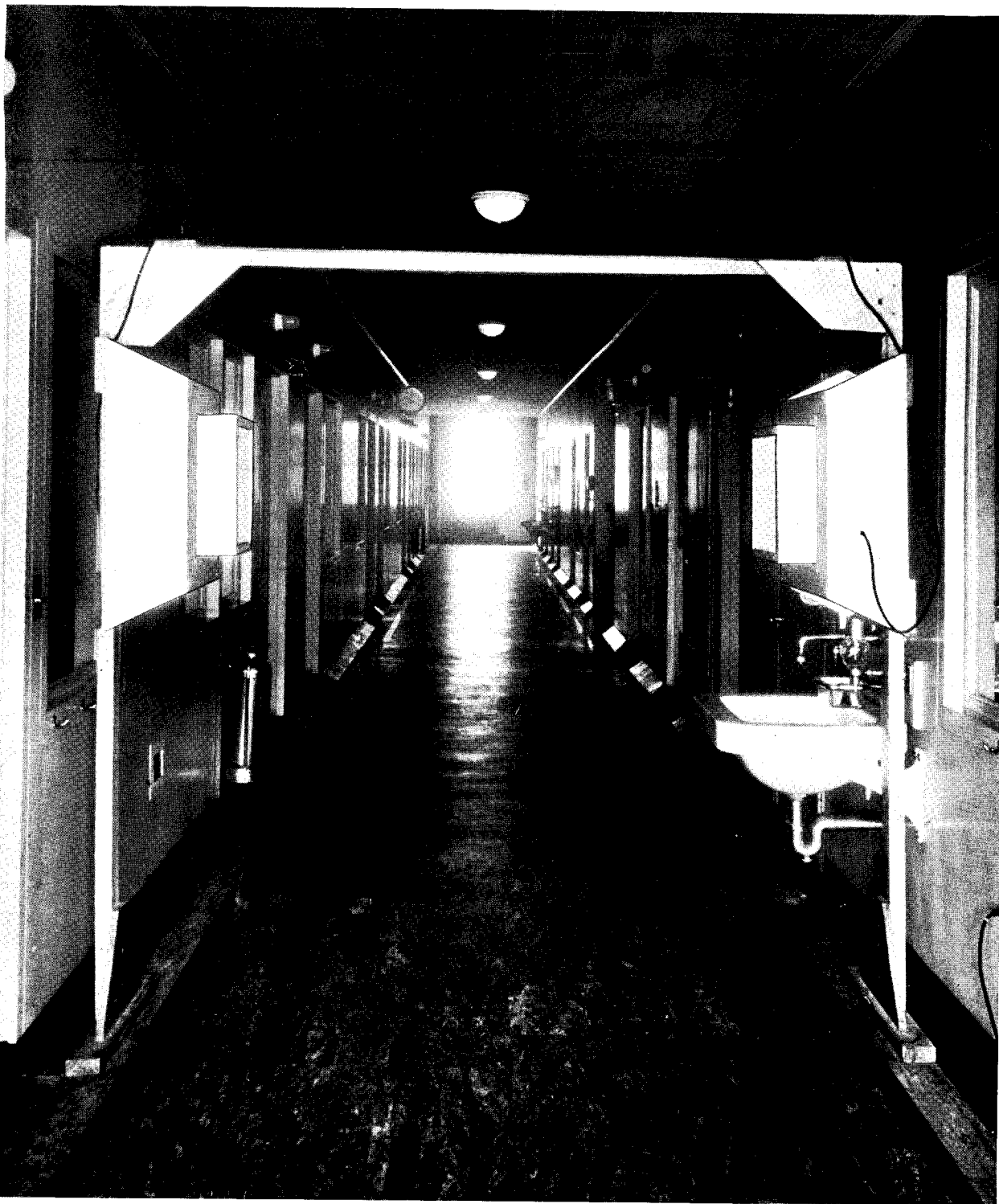
A barrier of ultraviolet light across the corridor of the isolation unit of the Children's Hospital in Boston, Massachusetts. Tests have shown that such screens can be made practically impervious to air-borne bacteria.
