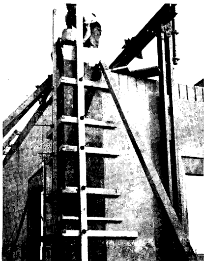
"Tilt-up" construction; entire walls are cast as units on poured first-floor platform, raised, and joined by poured corner-posts.
