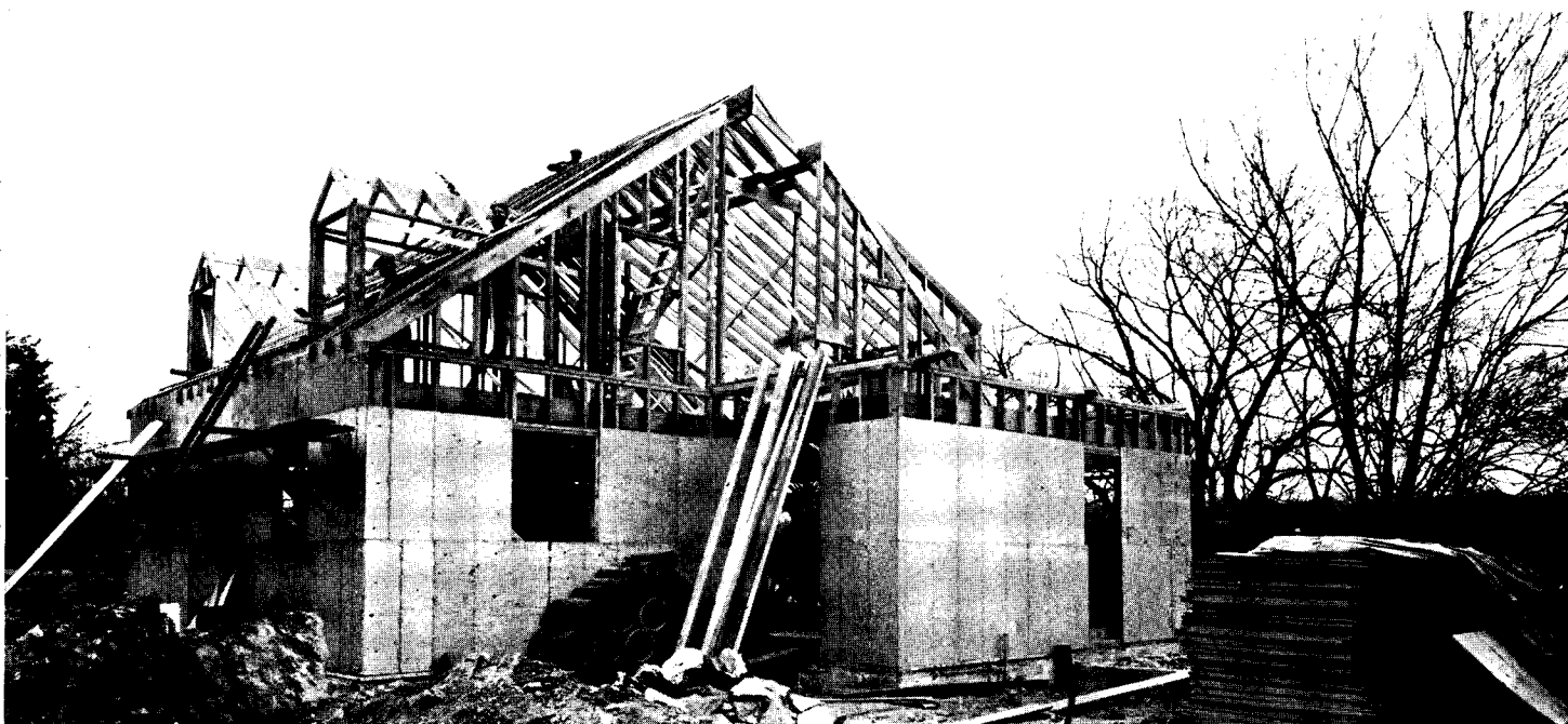
Photographs on these two pages record construction of a typical small house built in Stamford, Conn., for R. B. Edward. Richard Everett was the architect. Important is the fact that, built by a typical residential contractor, the conventional finished product contains plywood subflooring, sheathing, and interior finish.
