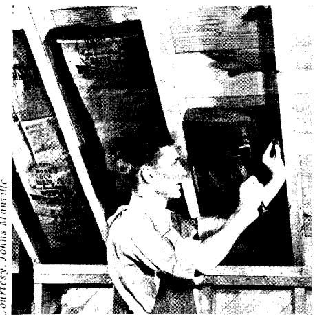
Tacking-flanges on wool-batt and reflective-metal types of insulation simplify installation.
