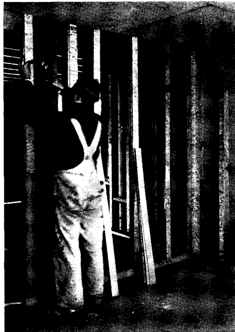
Applying "Furstix" (sanded 1/4-in. plywood cushion strips) to studs, to receive interior plywood.
