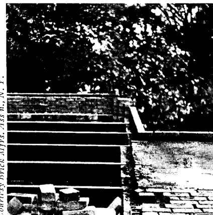
Reinforced brick floor panels between steel joists are a comparatively new development.
