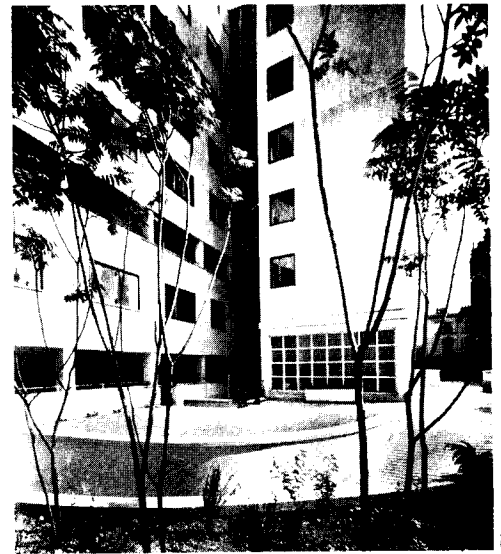
Entrance front, showing exit from garage.
