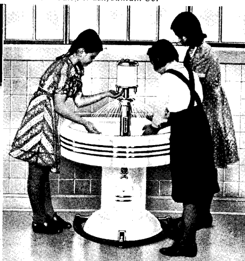
is minimized by the use of treadle-operated group-washfountains and . . .
