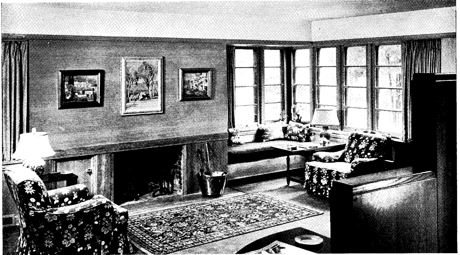
Living room, from entrance hall. Plywood on walls is quarter-sawn white oak. Plaster has silica sand-floated finish.
