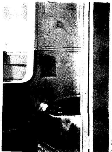
A bathroom designed by R. Buckminster Fuller; 5 by 5 ft., its total weight is about one-quarter that of usual bathrooms.
