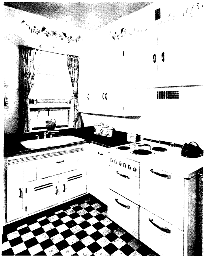
Typical kitchen: specially-designed cabinets incorporate electric range and refrigerator; counters are finished in Masonite, floors in linoleum. All ranges are vented by forced draft.
