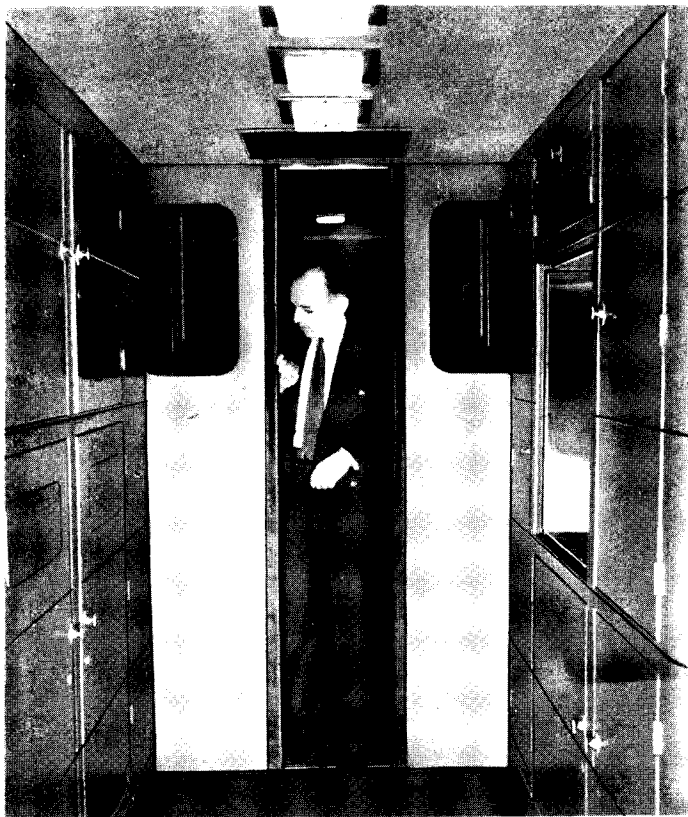
When the time-delay relay clicks, the doors start to close but reopen at a touch of the sensitive edges of the doors.
