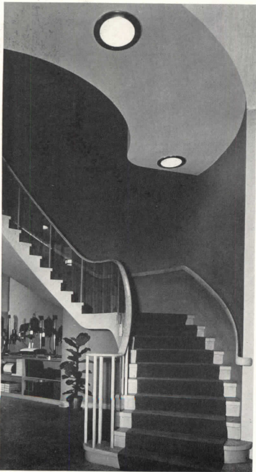
Cantilevered stair to the second floor
