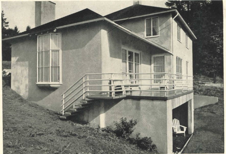
Detail of cantilevered balcony and stair leading from terrace. Uprights of the balustrade are of 1½-in. pipe, which have been drilled to support wood rail dowels.
