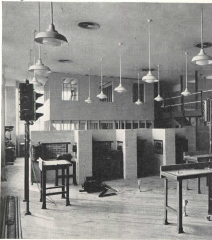
Built-in provisions for electrical work in South Vocational High School, Pittsburgh, Pa., include two types of booths, underfloor power service, a partly built house.
