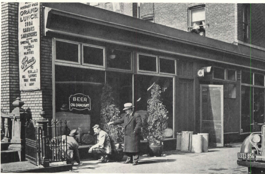
In the field, F. Treffeisen and J. Olson plan the procedure of a remodeling job.
