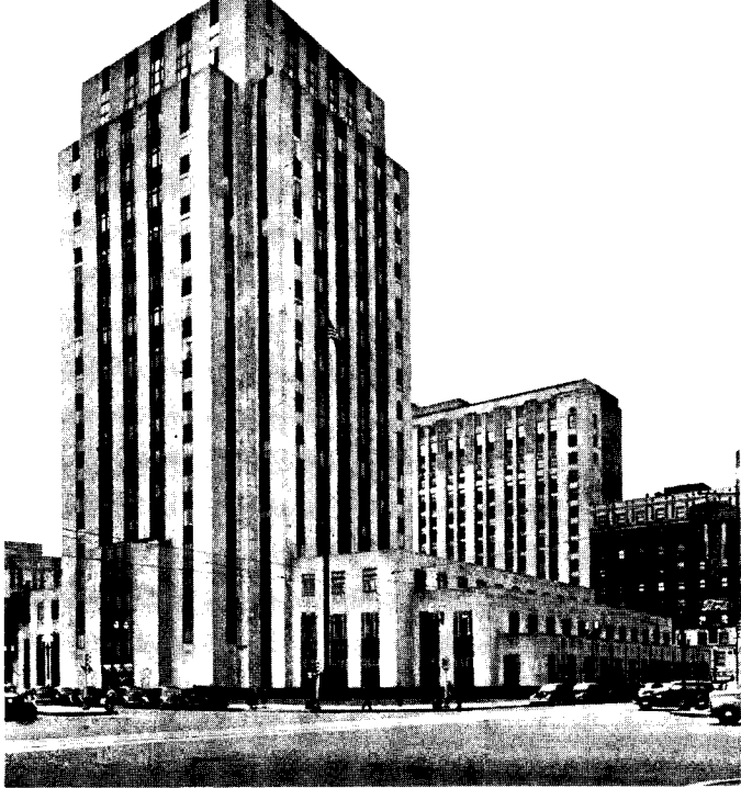
SEVEN VOTES: The St. Paul Courthouse, by Ellerbe and Co., Architects; Holabird and Root, Consultant Architects.
