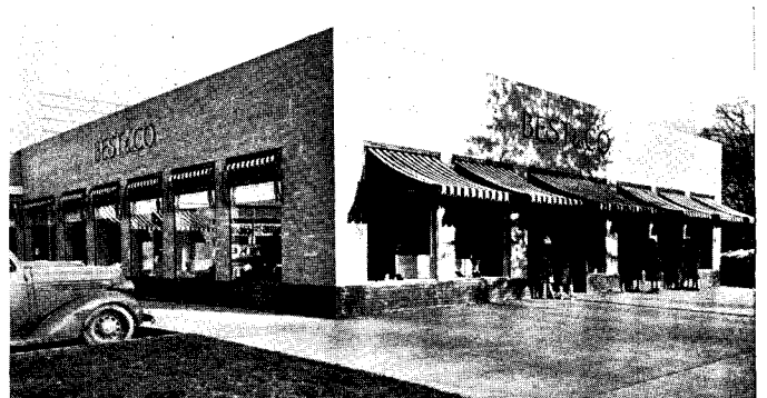
One of the 1-story wings contains a branch department store.
