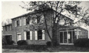
West Dodd also installed the lightning protection system on the Fire Safe House sponsored by the Home Insurance Company and featured at the New York World's Fair.
