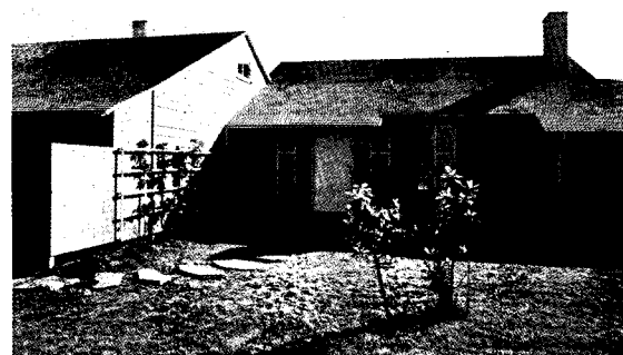
Entrance, with garage and auto court at left
