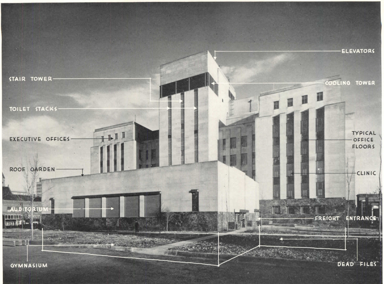
ARTHUR H. NEUMANN & BROTHERS, Inc., General Contractors; CHARLES S. LEOPOLD, Heating and Air-Conditioning Engineer; B. E. LANDES, Mechanical Engineer for Plumbing and Electric Wiring; DR. PAUL E. SABINE, Acoustical Engineer
