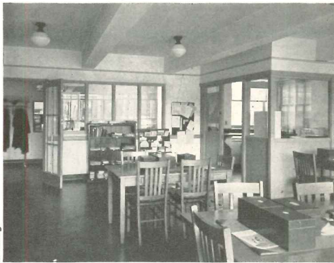
Demountable partitions increase flexibility.
