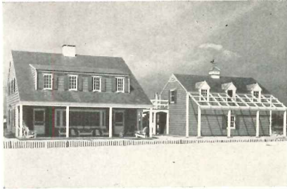
Cabot-Stained house, Beach Haven, N. J. Architects: Savery, Scheetz & Gilmore, Phil.
