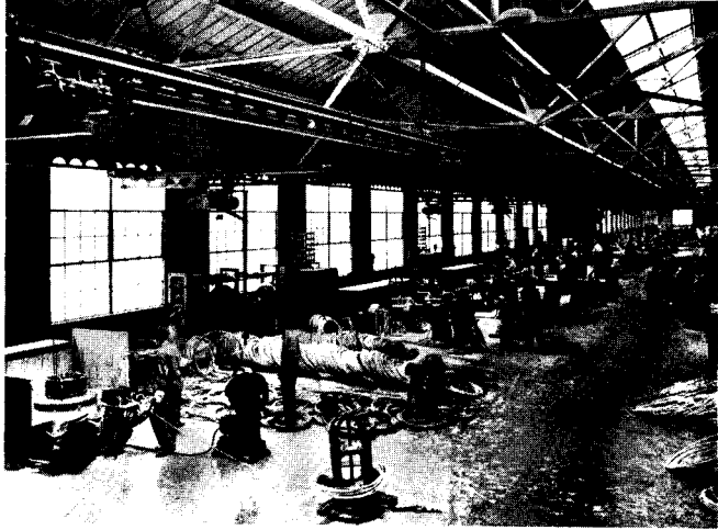
Suspended conveyors add to truss load
