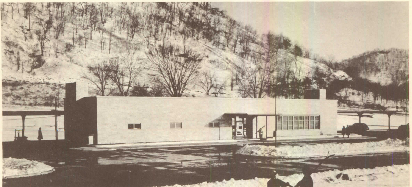
LA CROSSE, WIS. Station for the Burlington Road. Holabird and Root, Architects
