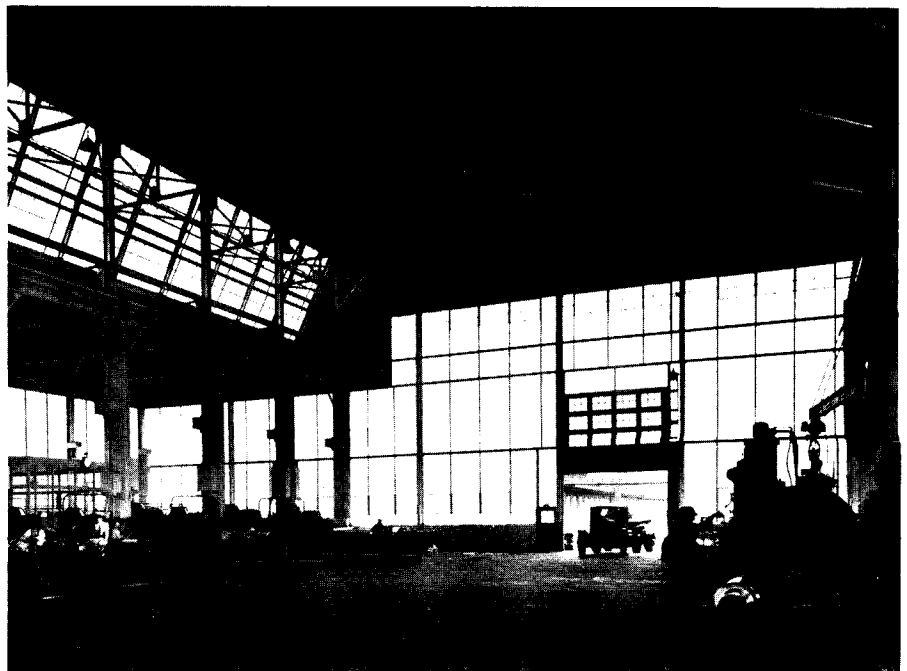
Wide spans, emphasized in the tremendous center bay, permit utmost freedom in layout of plant processes: shifts in production flow can be made without restraint. Notice the suspended directional unit heaters.
