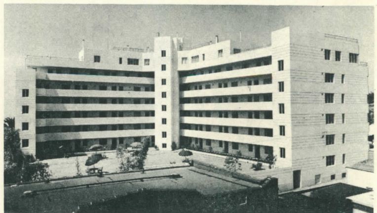
FROM GARDEN SIDE (garage under)
