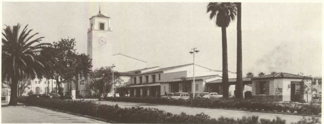
GENERAL VIEW showing parking area in foreground
