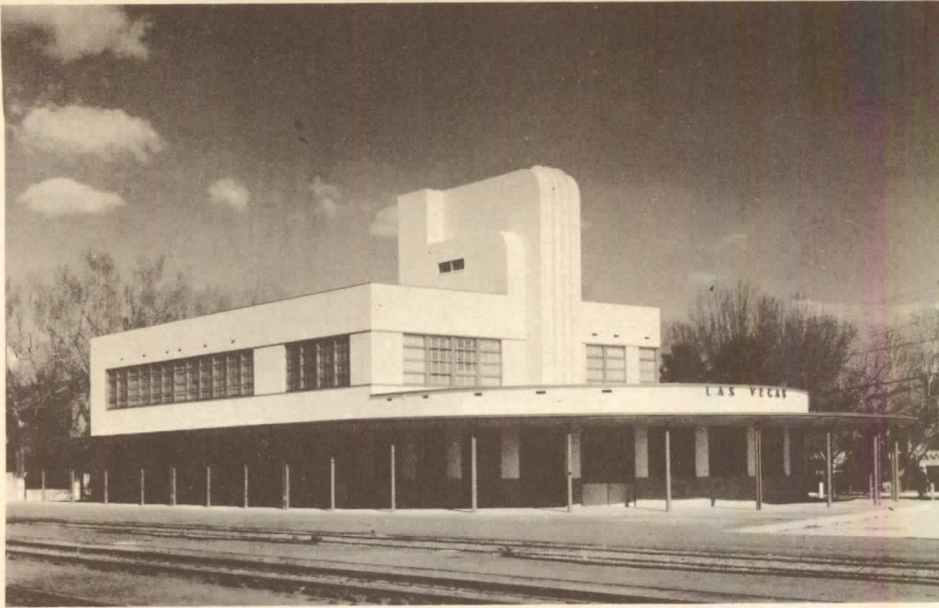
LAS VEGAS, NEV. Station for Union Pacific Railroad. H. L. Gogerty, Architect
