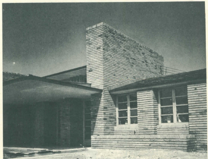
ENTRANCE DETAIL, north side.
