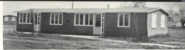
One-story double house, by FSA at Ceres, California
