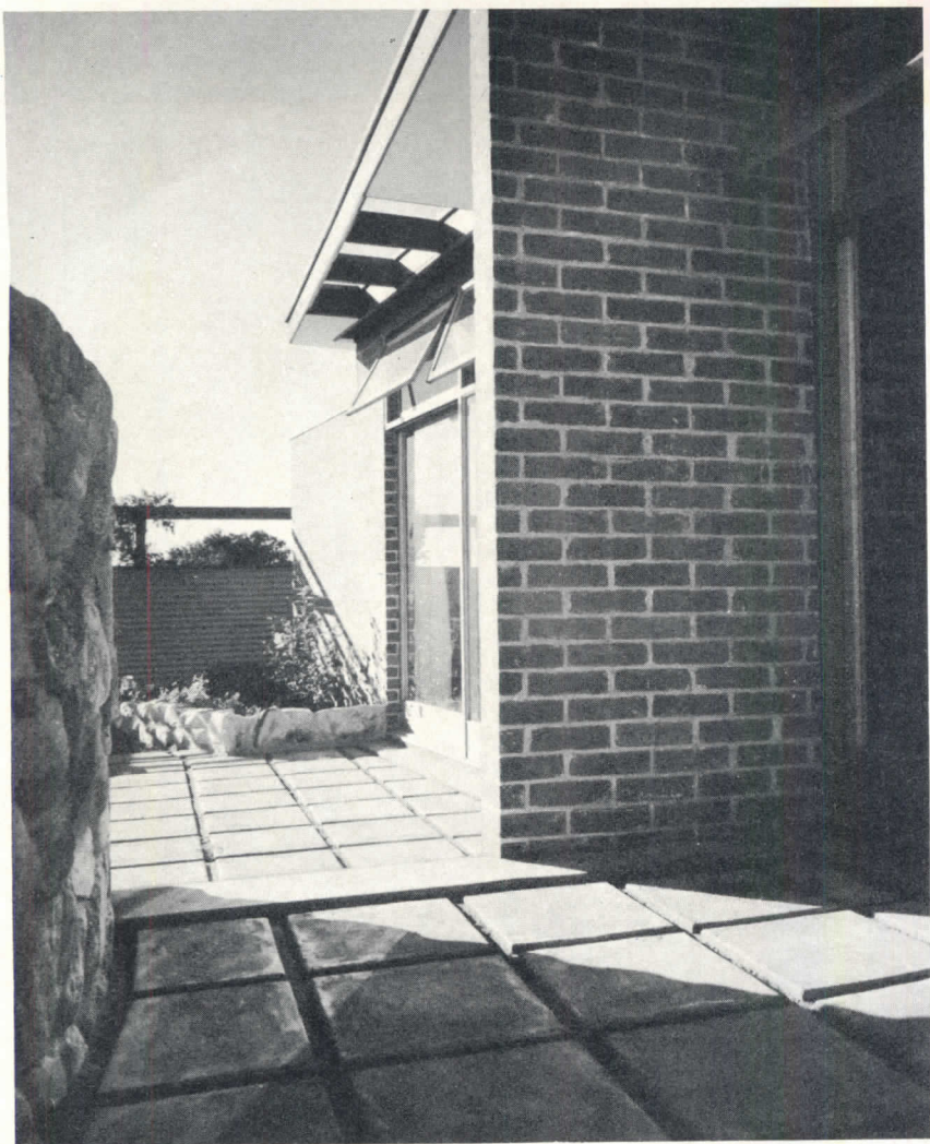
TERRACE: looking from bedroom toward living room
