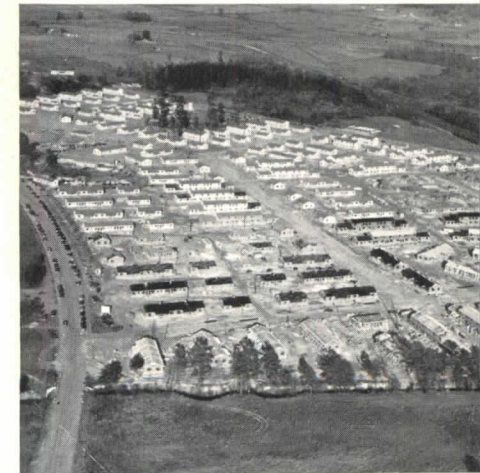
Newton D. Baker village, Columbus, Ga., USHA-financed, for families of noncoms at Fort Benning; L. D. Haines, Chief Archt.
