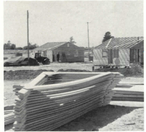
Standardized mass production on the site, for FSA farm homes, unimpeded by building codes
