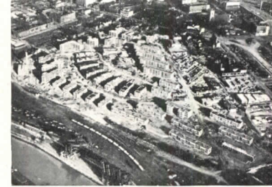
Lakeview Terrace, Cleveland, O. (PWA)
