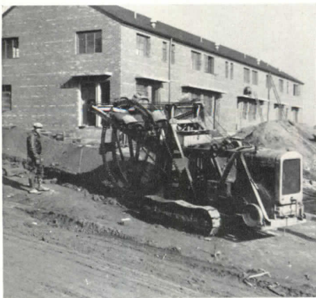
Rationalized and mechanized USHA job operation: excavation by mechanical trench diggers
