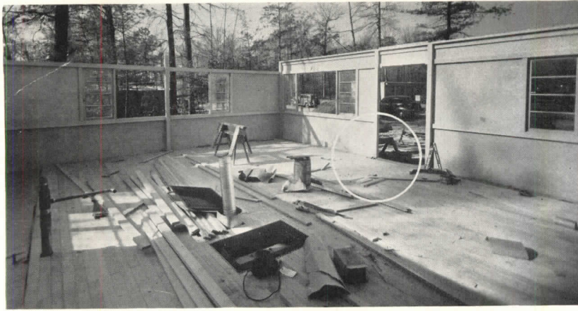
Interior view of wall elements in place
