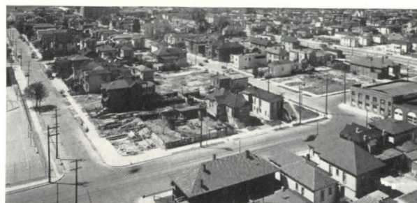
BLIGHTED: Site of Peralta Villa, Oakland, Calif.
