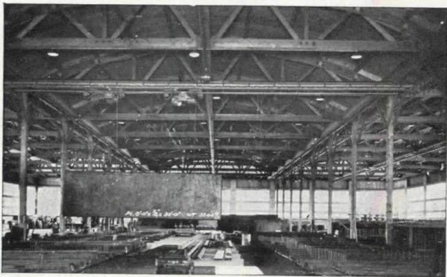
PORTLAND. Steel warehouse for Woodbury & Co. The roof of this 200'x300' building is supported by 35-67' trusses, 15 lb. dead load, 40 lb. live load, plus 14,000 lb. concentration at center line of bottom chord and adjacent to each end of the truss. Concentration supports a three-point suspended traveling crane. Architect: Richard Sundeleaf. Contractor: Wegman & Son.
