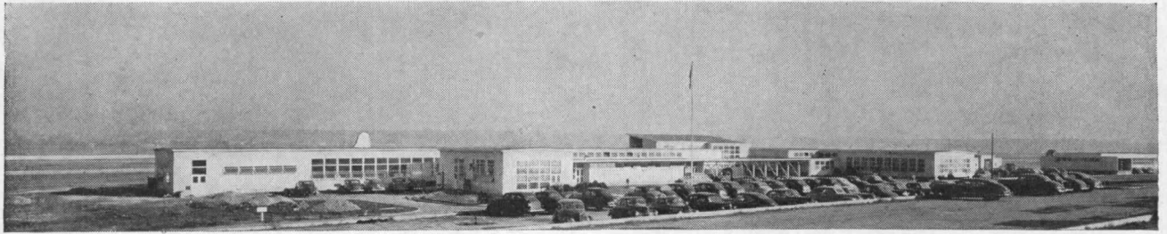
ATC's Washington terminal is based on 16-ft. unit bays, subdivided into three 5 ft. 4 in. design units
