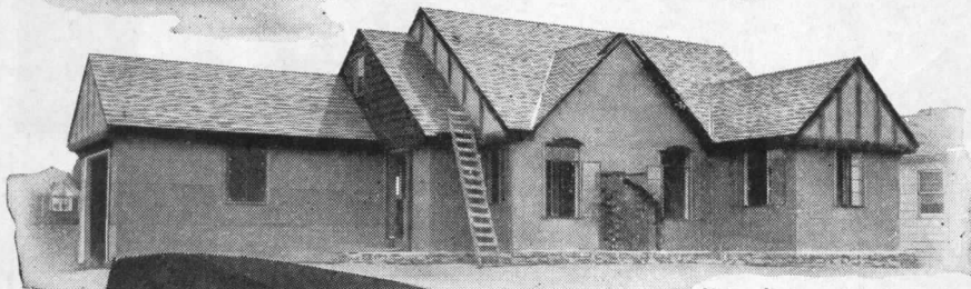
Note absence of batten strips and tears in this SISALKRAFT application. This reinforced paper is strong enough to pull around corners.
