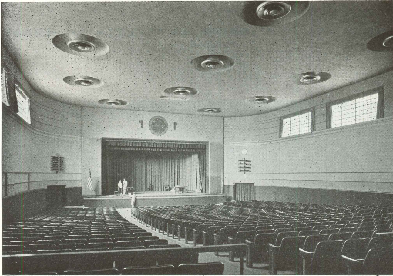
Anemostats diffuse warm air and contain lights. Dado is hard wallboard; walls, acoustic plaster; ceiling, sand-finished plaster
