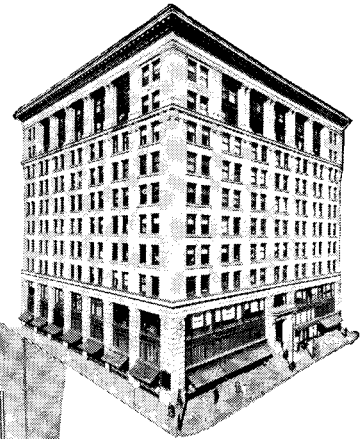
Slater Building, Worcester, Mass.
