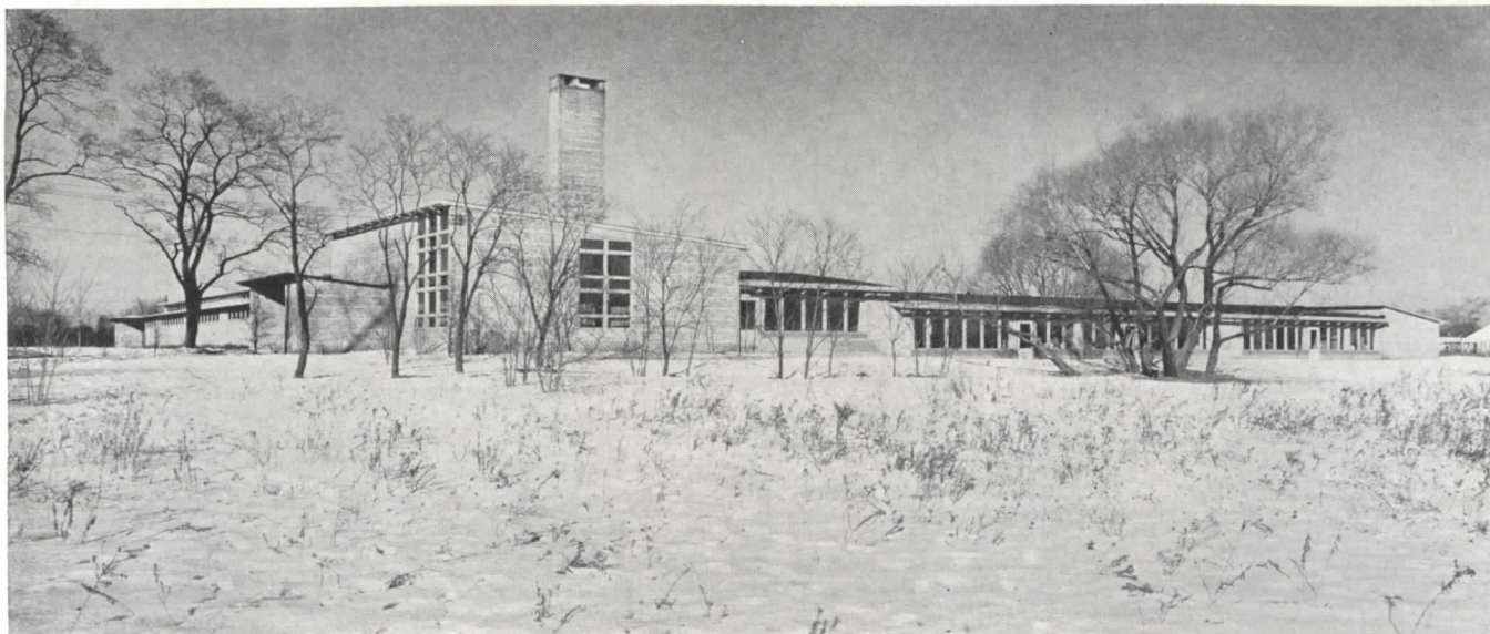
The Rugen School, Glenview, Ill.; Perkins, Wheeler and Will, architects. The firm had some 30 schools on its boards at presstime
