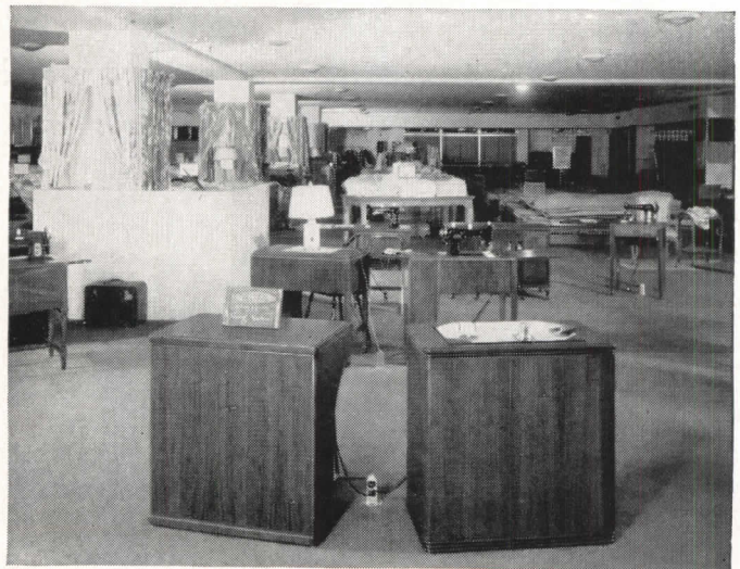
Above photograph is of a sales floor in a store with G-E Q-Floor Wiring. Note the many floor outlets in different parts of the room. Power is readily available for working models, etc.
