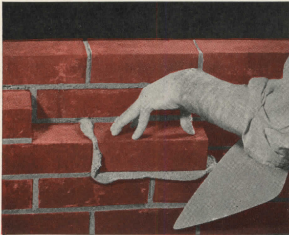
To compare the plasticity of any two mortars, try shoving a brick into place, with a full head
