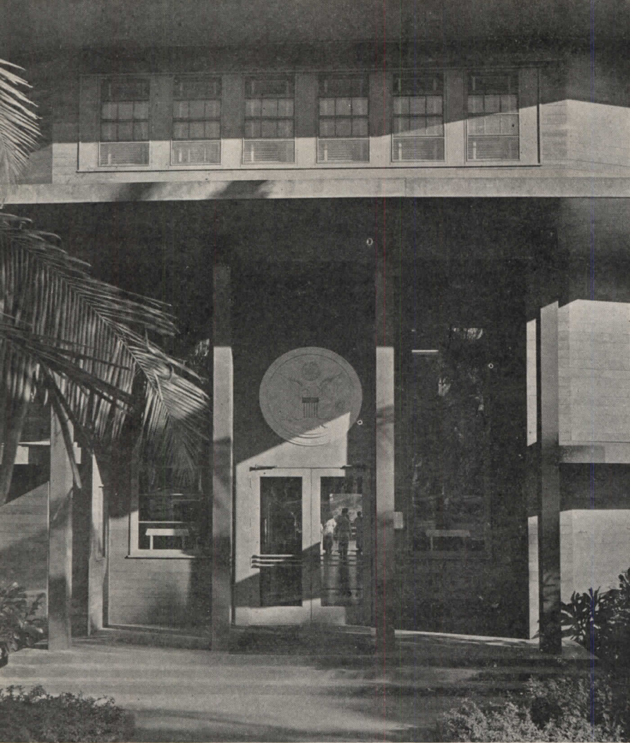
Left: Main entrance to Building "A" has two-story wood columns and recessed lanai. The great seal of the United States is made of built-up plywood finished with aluminum paint. The lobby opens to the main passage to Building "B". Left below: main entrance lobby of Building "A". Fluted columns are painted a rich blue-green. The mural was designed by Master Sergeant William R. Domaratius. Site conditions at the entrance, and the road elevation in front of the building, made it necessary to keep the entrance high to prevent having the building appear to be down in a hole. The lobby floor was therefore raised two steps above the rest of the first floor. Center: this view of the Commanding General's office shows the plywood wall finish, asphalt tile floor and acoustical ceiling. Fluorescent lighting is recessed in a 6-in. furred space in the ceiling; this space is available throughout the building for the complicated communications wiring. Right below: main axis corridor from lobby of Building "A" to third floor balcony of Building "B"
