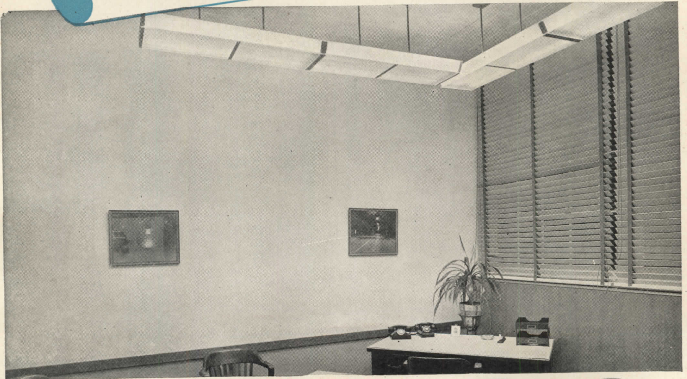
An ideal layout for an office of this type, using four type LW-160 Luminaires.
