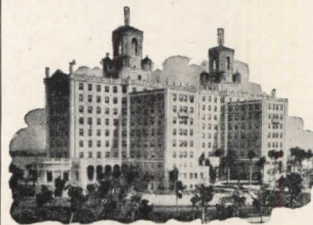
The National Hotel at Havana uses Frick Refrigeration for half a dozen services.
