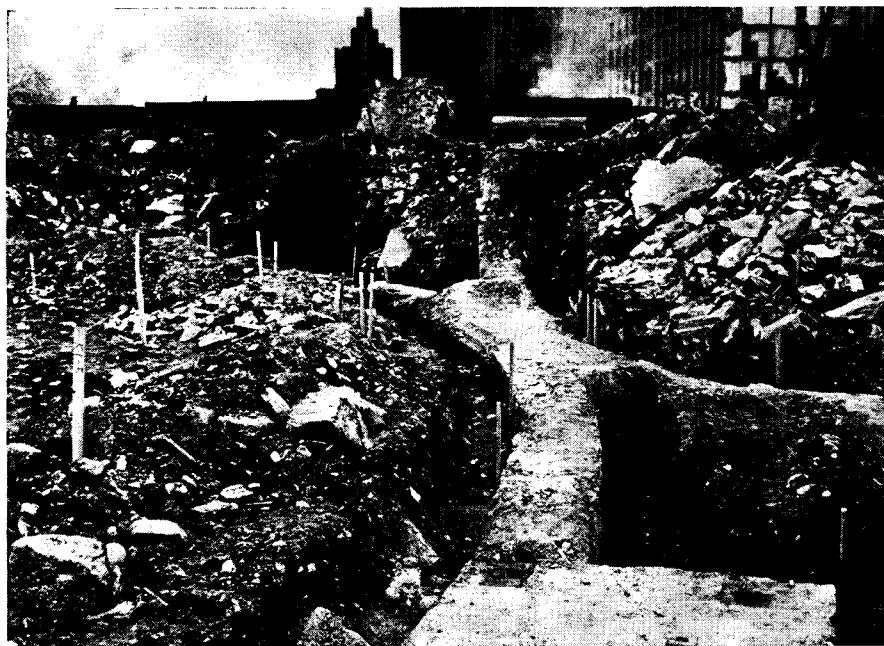
Old, hidden foundations of demolished gas tanks necessitated special pile-driving operations at Stuyvesant Town site. Beneath broken stone rip-rap lies concrete floor, 2 ft. thick
