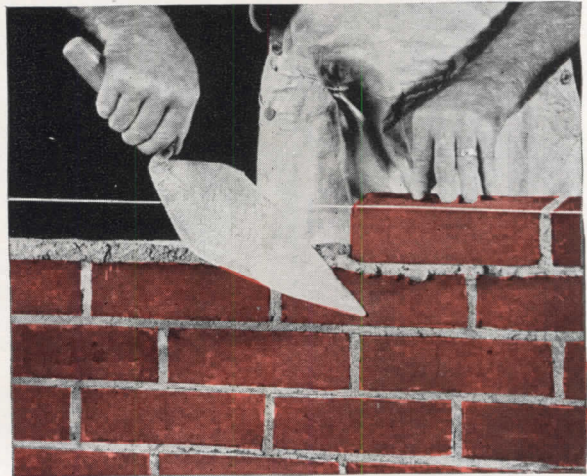
two photographs above show a good comparative test for plasticity—hence for bond. Try this with Brixment mortar!
