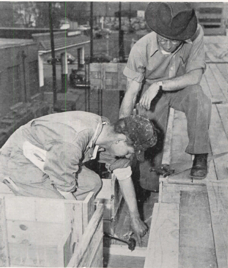
After a little interruption of three and a half years, spent in the Army Air Force, Melvin T. Brody is back learning the carpentry trade, atop a new garage in Atlanta. R. W. Linsey, foreman
