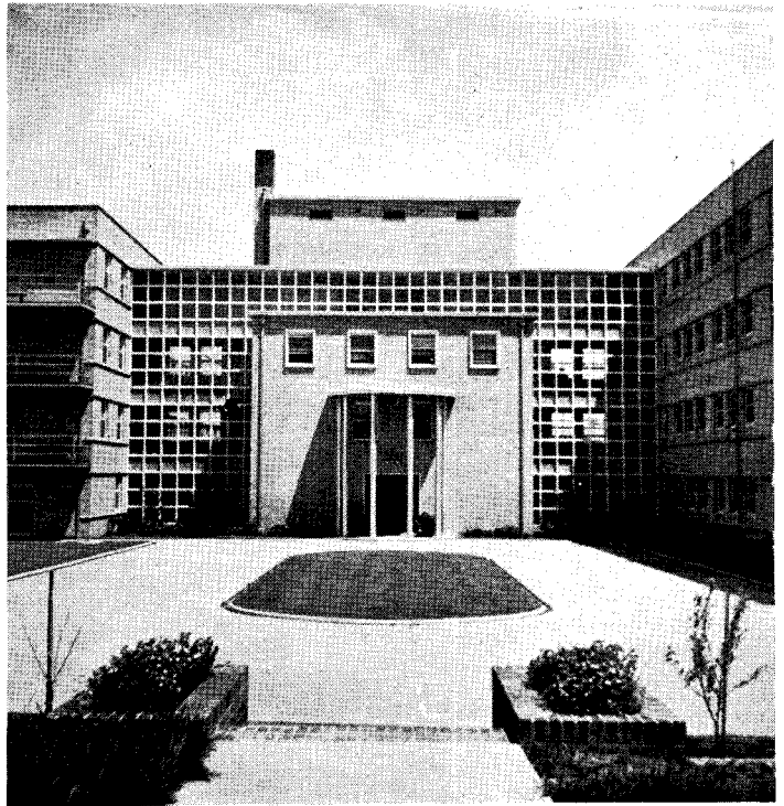
The Nurses' Home (right) also uses the system of prefabricated concrete frame, which lends itself to a variety of treatments — solid wall, windows, doors, ventilator or void
