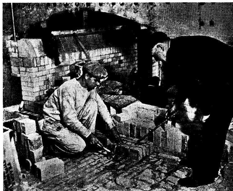
How to lay brick properly in a soaking pit floor is shown to apprentice Harry Floyd by H. D. Tyson, in a plant of the Tennessee Coal, Iron and Railroad Co. (U. S. Steel) in Birmingham, Ala.
