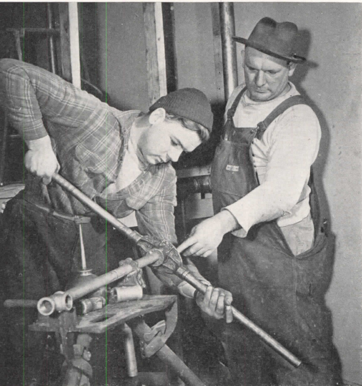
The tradition of craftsmanship is here being carried on by a father-and-son team. Journeyman plumber John E. Grove of Washington, D. C., shows John G. Grove how to thread a pipe
