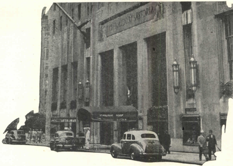
Park Avenue entrance to The Waldorf-Astoria, New York. Anaconda Architectural Nickel-Silver, fabricated by the General Bronze Corporation, Long Island City, New York, is used extensively at entrances and doors. Architects: Schultze and Weaver; (now Leonard Schultze & Associates), New York.
