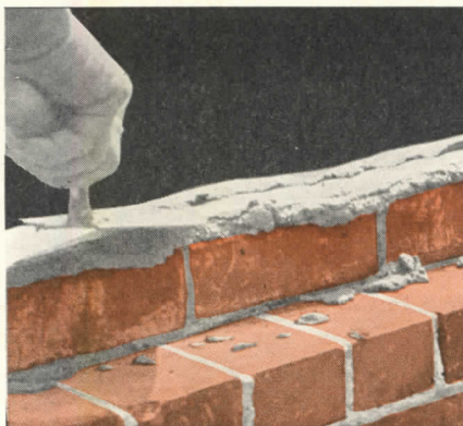
The furrow in the mortar should be shallow, not deep.
