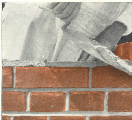
A thick bed of mortar should be spread on the wall.
