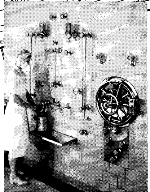
SCANLAN-MORRIS Recessed Water Sterilizers and Autoclave
