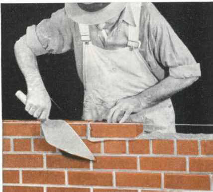
So the mortar will still be soft and plastic when the brick are bedded.
