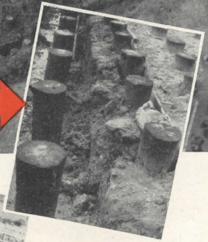
Piles in trench will be capped by wall; others by floor slab.
