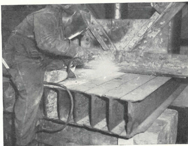
Fig. 1. Welding bottom of truss to needle beams acting as temporary support.
