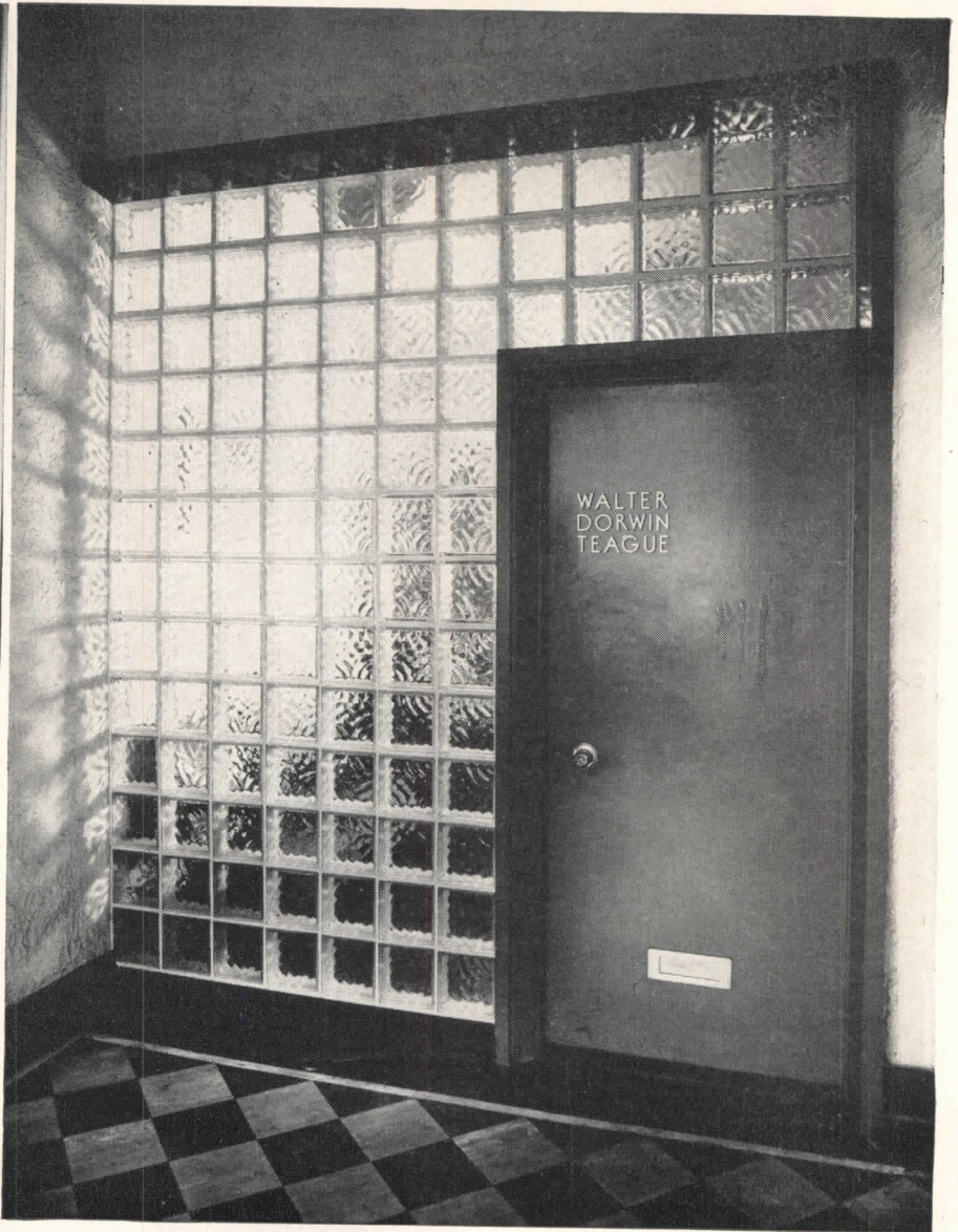
Insulux partition provides privacy in reception room of Walter Dorwin Teague's Los Angeles office—adds daylight and more spacious appearance.
