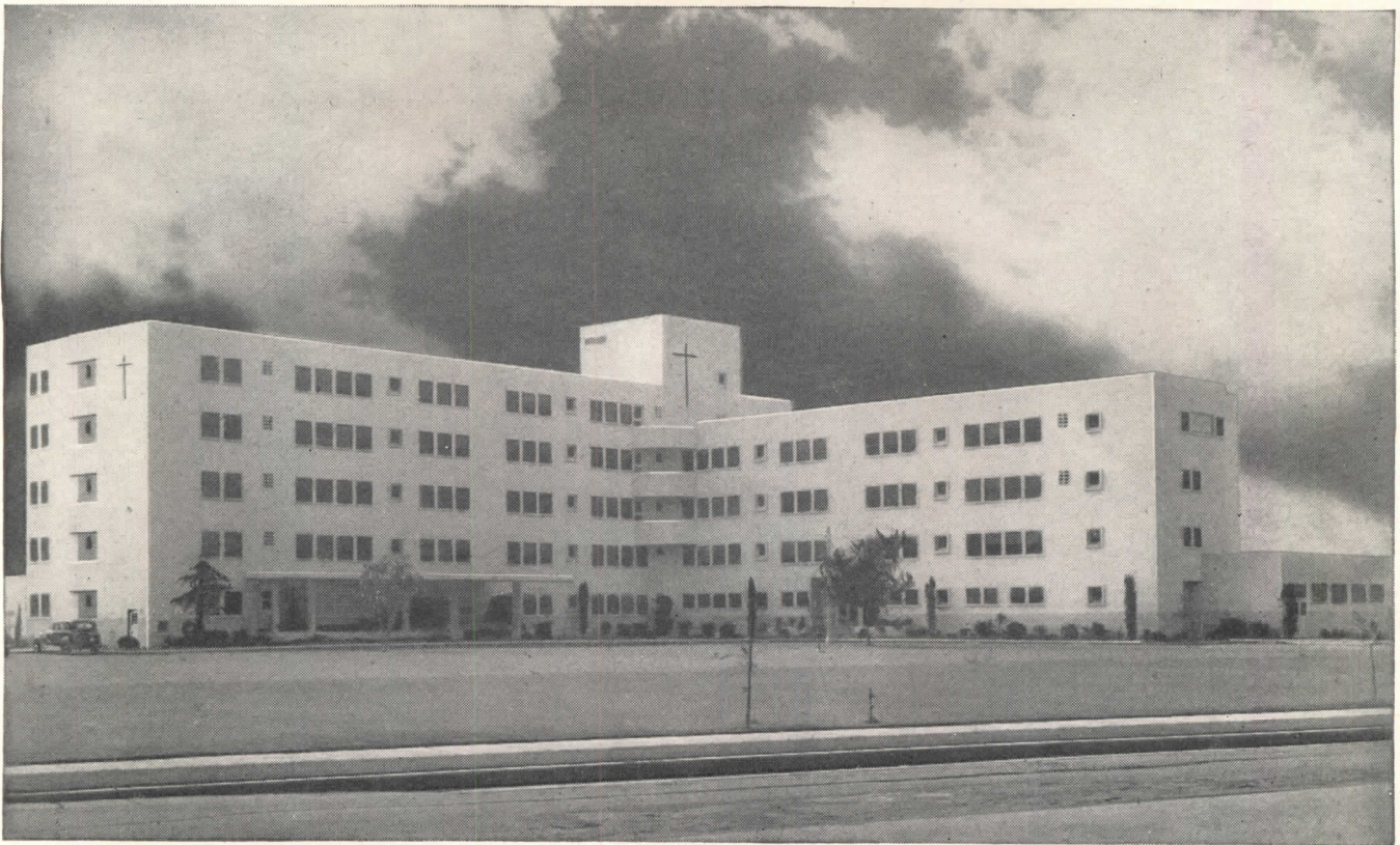
St. Francis Hospital, Lynwood, California. George J. Adams, architect; Hillman & Nowell, structural engineers; Thomas & Beyer, general contractors.
