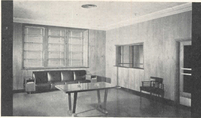
Walls of the first floor lobby, left, are in natural walnut veneered hardboard. Walnut and red leather upholstered furniture throughout the building was especially designed by The Austin Co.
