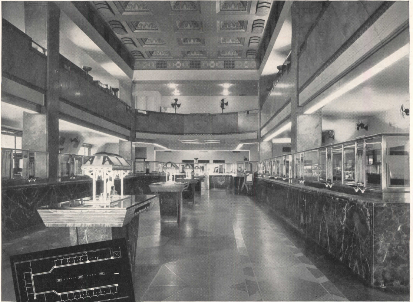
Manufacturers Trust Co., New York City. To furnish 40 foot candles in tellers' counters from fixtures to blend with existing decor, continuous sections of 40W incandescent lamps with individual reflectors and No. 739 Holophane lenses were mounted on the soffit over the counters. Finish is sprayed bronze.
