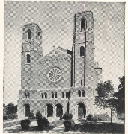
CHURCH OF THE MOST HOLY ROSARY, Syracuse, N. Y., N. H. LaVaute, Architect. M. B. Moyer, Consulting Engineer. Modernized 1946 with Webster Moderator System of Steam Heating. Joseph Burke, Heating Contractor. Hillebrand & Owen, Electrical Contractor.
