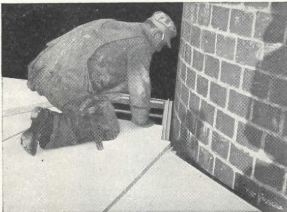
KAYLO INSULATING ROOF TILE can be cut and fitted with ordinary hand or power tools right on the job.
