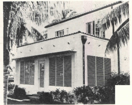
Plexiglas jalousies in a variety of colors serve as awnings and storm shutters
