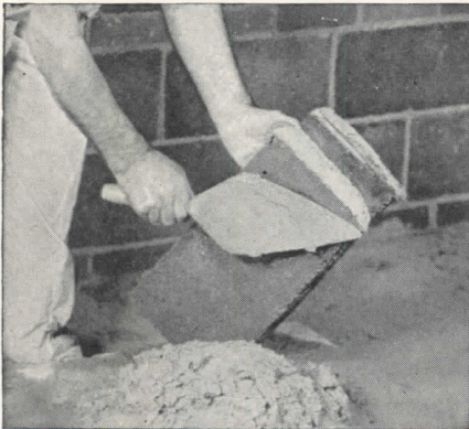
Method 1. Full head joints should be thrown onto both edges of the block to be placed, or—
