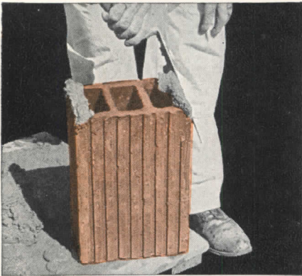
Method 1. Full head joints should be thrown onto both edges of the tile to be placed, or—
