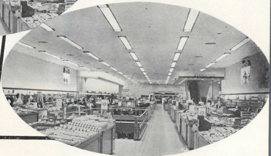
d: Cove lights plus general fluorescent plus incandescent inserts: Results: a perfect combination of lighting for selling.
