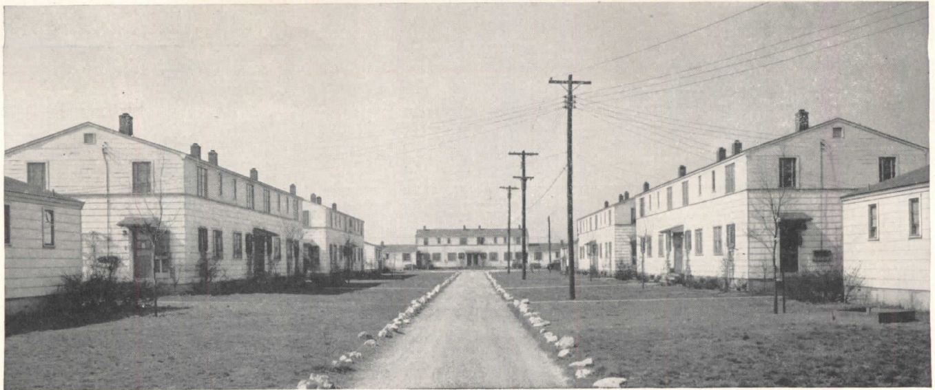
This Indiana housing development features "Century" Asbestos-Cement Siding on first stories, with K&M "Century" Apac board used as skirting at the foundations.
