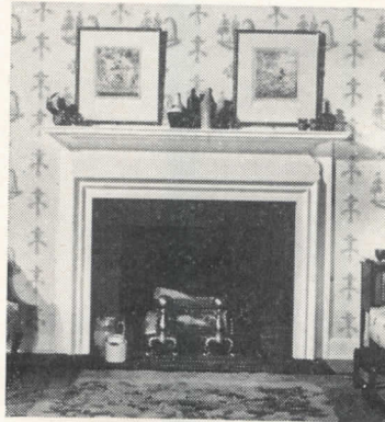
A late eighteenth century mantel—adapted from one in the old Lee House at Marblehead, Mass. Note the unusual shape of the fascia board. Fits any traditional style architecture. Design C-6063.
