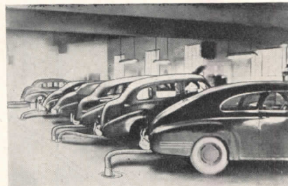
Car exhaust is fed through flexible tubes to floor ducts and then vented outside
