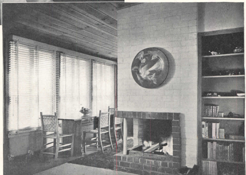
Floors throughout are colored cement on concrete slab. Except in kitchen and bath, ceilings are V-jointed pine boards, oiled and waxed. Walls are painted
