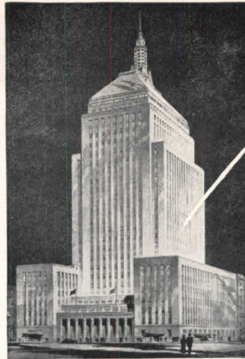
John Hancock Mutual Life Insurance Co. office building, Boston, Mass. Cram and Ferguson, Architects. Turner Construction Co., Contractors.
