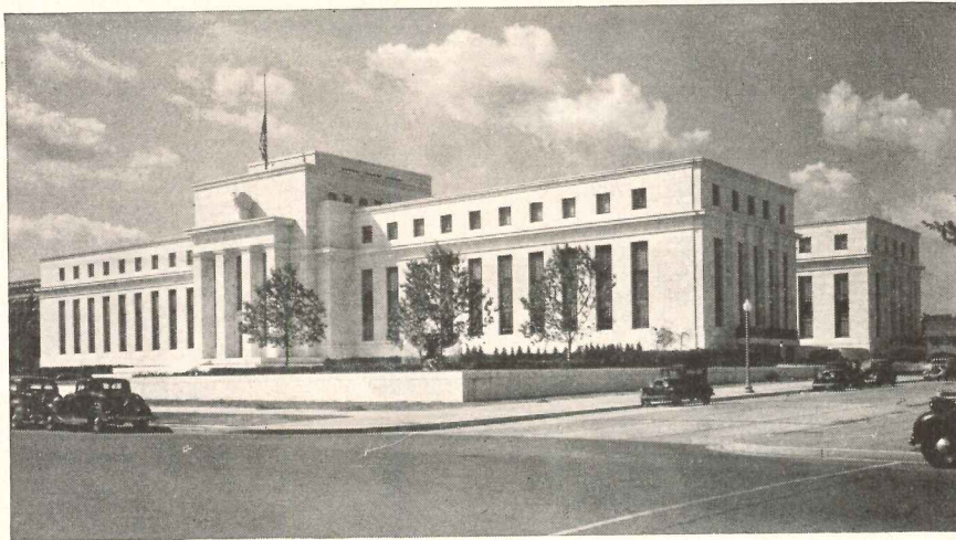
Federal Reserve Building, Washington, D. C. Paul P. Cret, Architect, Philadelphia, Pa. George A. Fuller Co., Contractors, Washington, D. C.
