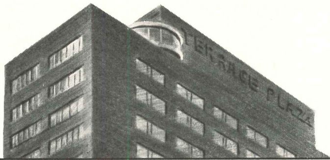
Terrace Plaza Hotel, Cincinnati, Ohio, in which some 135,000 pounds of Revere Copper Water Tube were installed.
