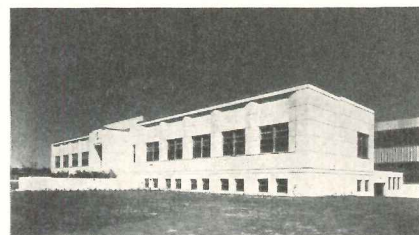
Plant for Turner-Newall (Canada) Ltd., at Montreal covers 10 acres, is devoted to manufacture of asbestos products. Designed by E. C. Miller of T. Pringle & Son Ltd., consulting engineers.
