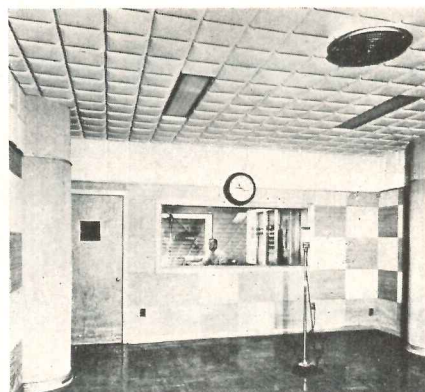
Cotton acoustical tile in radio studio
