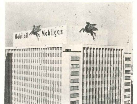
Enameled iron pans sheathing steel roof structure (above) match terra cotta building (below) and achieve reduction of dead load to \frac{1}{6} - \frac{1}{7} of terra cotta weight
