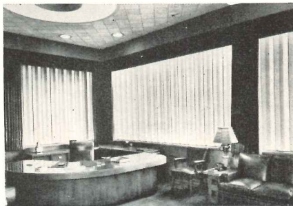
Metal jalousies provide sunlight control
