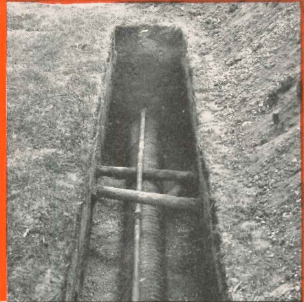
1941: Asphalt-coated conduit still in perfect condition.
