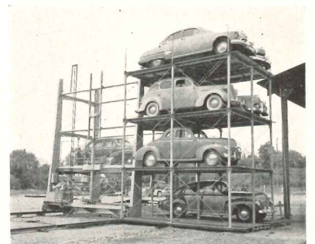
Cars are stacked four deep in steel racks
