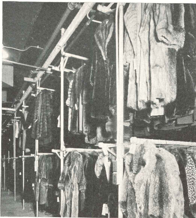
Proper spacing of furs in the vault is essential for good ventilation. (Photo courtesy Abbott, Merkt & Co., Engineers)
