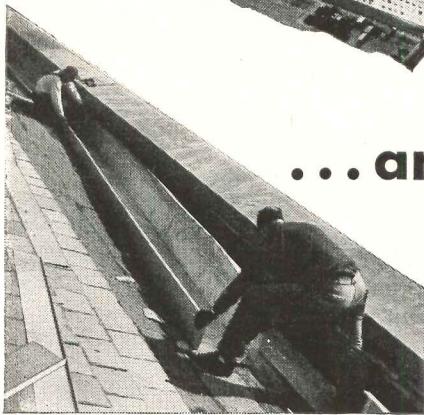
INSTALLING A RIVETED AND SOLDERED section of Monel Roofing Sheet in the built-in gutter of the Pentagon's outer perimeter. Fabricator, Rupertus Sheet Metal Works, Washington, D. C., reports: "Some of the gutters were 55 inches in girth, but Monel was easy to fabricate and install."
