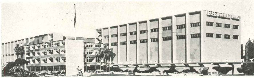
Lever Bros. processing plant at Los Angeles, Calif., leaves much equipment in the open
