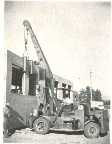
Crane hoists sandwich-type precast panels into place (above). Derrick is used with 16-in. panels of another system (below)
