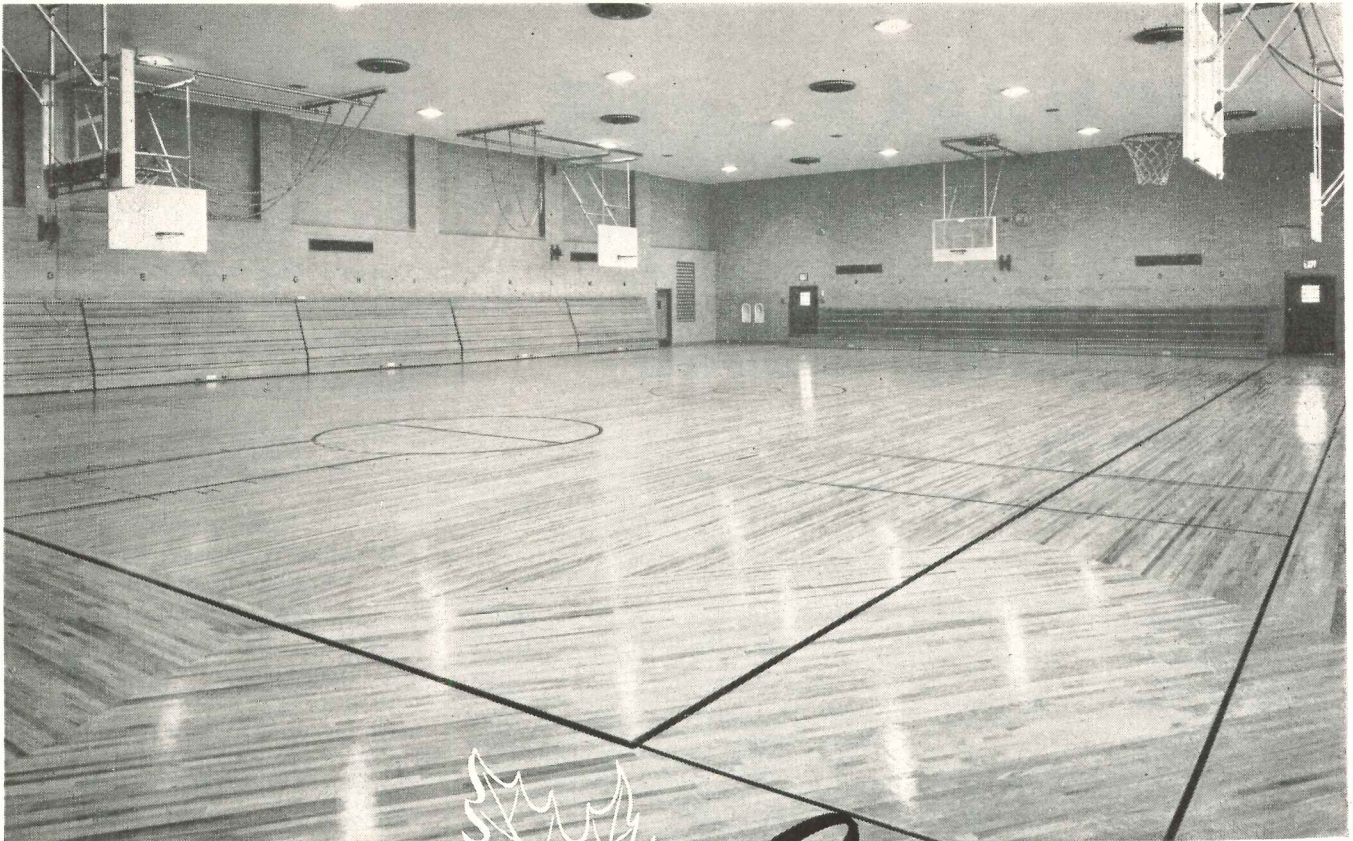
Floor of Northern Hard Maple, 80 x 100 feet, a dual-purpose innovation which combines gymnasium and roller-skating rink, at Archbishop Stepinac High School, White Plains, N. Y.—an interesting development in supervised recreation. Eggers & Higgins, Architects, New York, N. Y.
