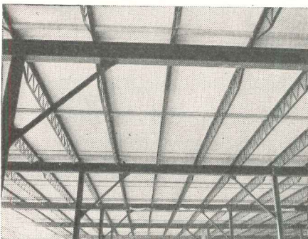
Light steel framing for 53,760 sq. ft. of Cemesto for Watson Terminal Warehouse Company, Youngstown, Ohio.
