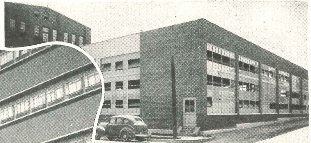
Truscon Commercial Projected Steel Windows with Rack and Pinion Operators, Century Ribbon Mills, Inc., York, Pennsylvania. I. Reindollar & Son, Inc., Contractor. Joseph D. Weiss, Architect.
