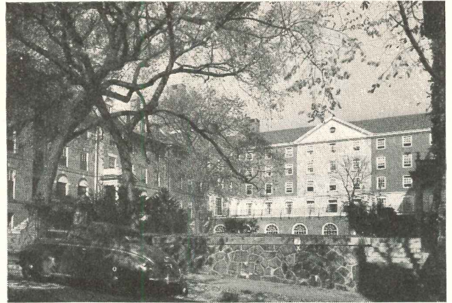
Revere Copper Water Tube in sizes under 2" and Red-Brass Pipe in sizes from 2" through 4" were used for plumbing lines in this new dormitory at PEMBROKE COLLEGE, Providence, R. I. Architect: Perry Shaw and Hepburn, Boston; Contractor: Joseph Cuddigan, East Providence, R. I.
