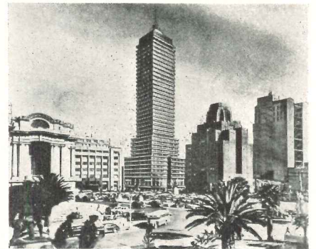
Mexico City's first 40-story building. By La Latino-Americana, Cia. de Seguros Sobre La Vida, S.A., engineering staff
