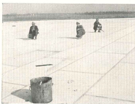
Caulking joints between Cemesto panels. Carolina Asbestos Co., Marshville, N. C. Contractor: Interstate Const. Co. Architect: A. G. Ulrey.
