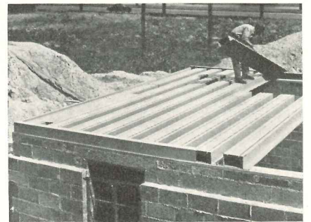
Structural floor serves as heat ducts
