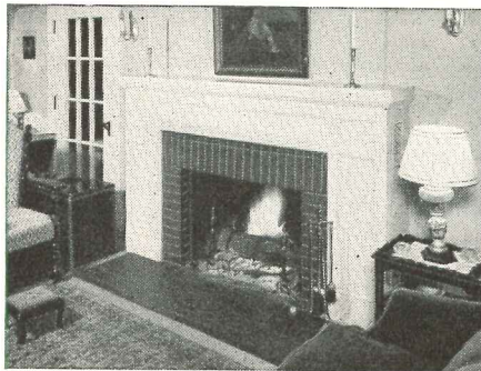
An example of warm air outlet grille placement in a fireplace with projecting mantel.
