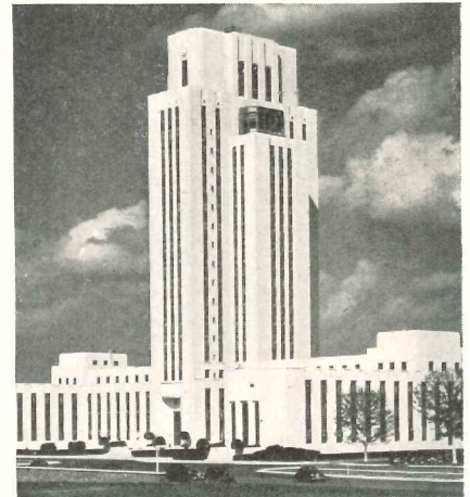
Naval Medical Center, Bethesda, Md. Minwax Weathercap used to protect masonry joints.
