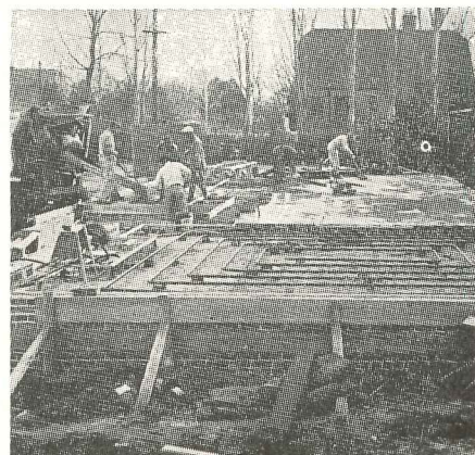
The inherent characteristics of steel pipe are perfectly "matched" to the installation requirements of Radiant Heating.
