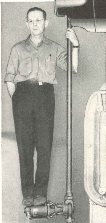
Illustration shows great strength of spring mounting which holds motor in perfect alignment always.
