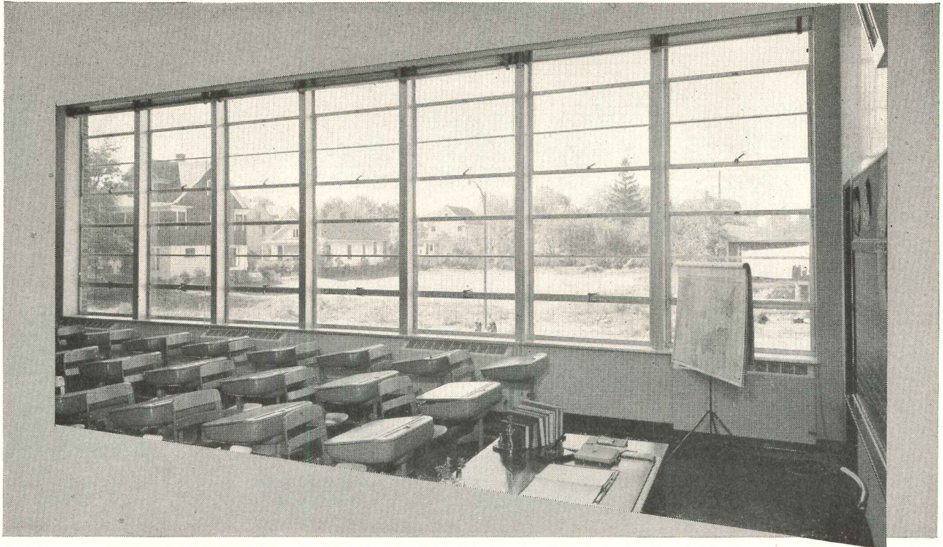
Architects Firestone and Lorscheider economically provided abundant daylight in St. Monica's School at Rochester, New York, with ceiling-high Fenestra Intermediate Projected Windows, light-colored Venetian blinds for light control, light-colored walls and ceilings to spread daylight.
