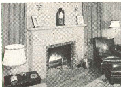
Typical placement of warm-air grilles in a projecting fireplace.
