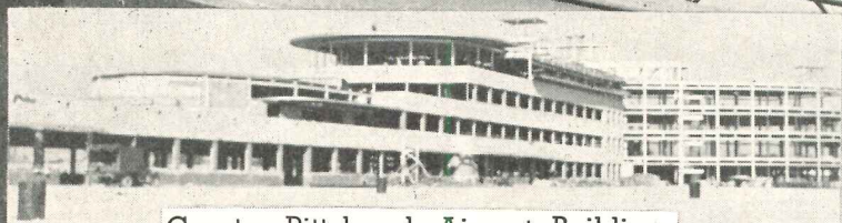
Greater Pittsburgh Airport Building
