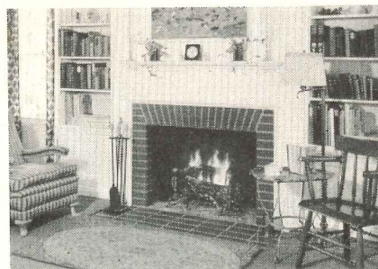
A Colonial Fireplace built around a Heatilator unit. Warm-air grilles are located in the bookshelf sides.
