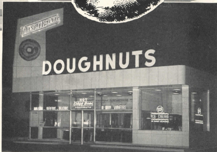
Thermopane Installation, Greensboro, N. C. Architect: Hall Crews, Winston-Salem.
