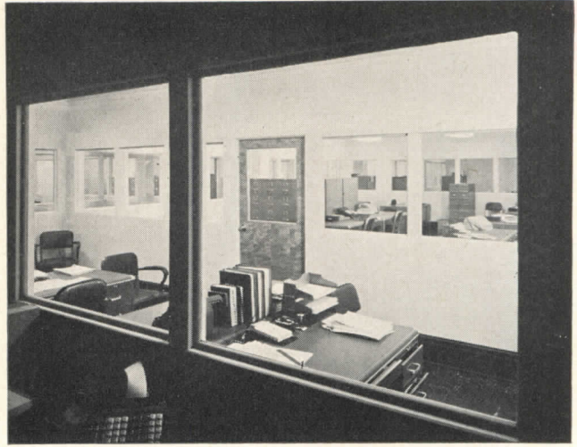
Left: conference room on second floor. The whole executive suite is paneled in Philippine Mahogany. Right: interior partitions are independent of metal tile ceilings to permit partition rearrangement
