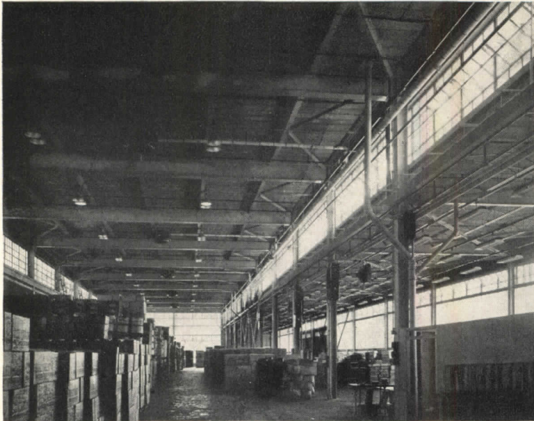
Detail at clerestory shows welded column-girder joint; roof bracing; rolled-section joists, widely spaced, over high bays; open-web joists over low bays where conveyors are supported. Below: section, sash and fixed corrugated wire glass in west wall
