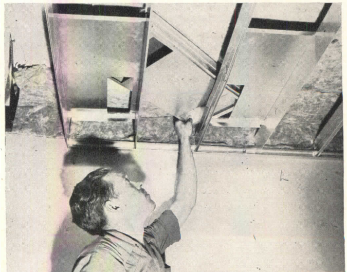
Installing the trough crossover
