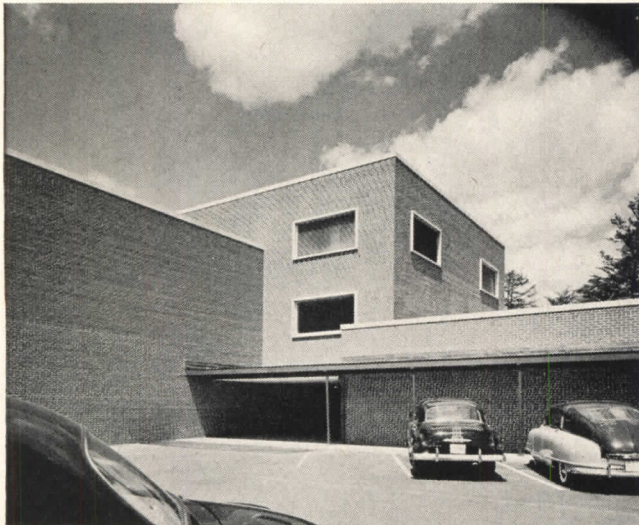
Equipment room has the only windows in the building, except for the ladies lounge, which is below it. In contrast to the Tide Water Building with its unit conditioners, the Stevens Building is heated and cooled by air. Cooling takes place in the equipment room, after which air is reheated by heating coils in the supply ducts to each zone so as to meet the variety of temperature requirements. The same coils furnish all heating
