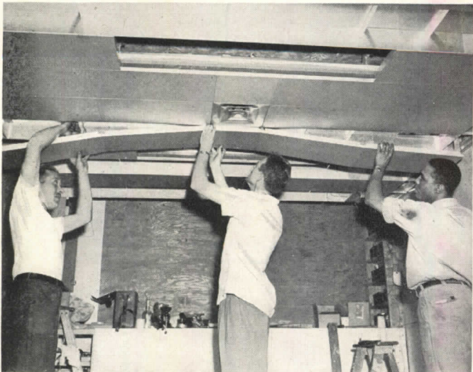
The ceiling air panel being attached
