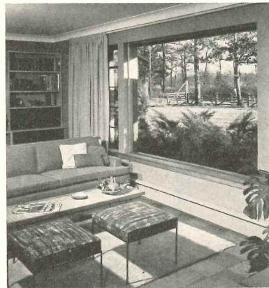
Baseboard convector projects only 1½ in. from wall. Units may be painted to match most color schemes.
