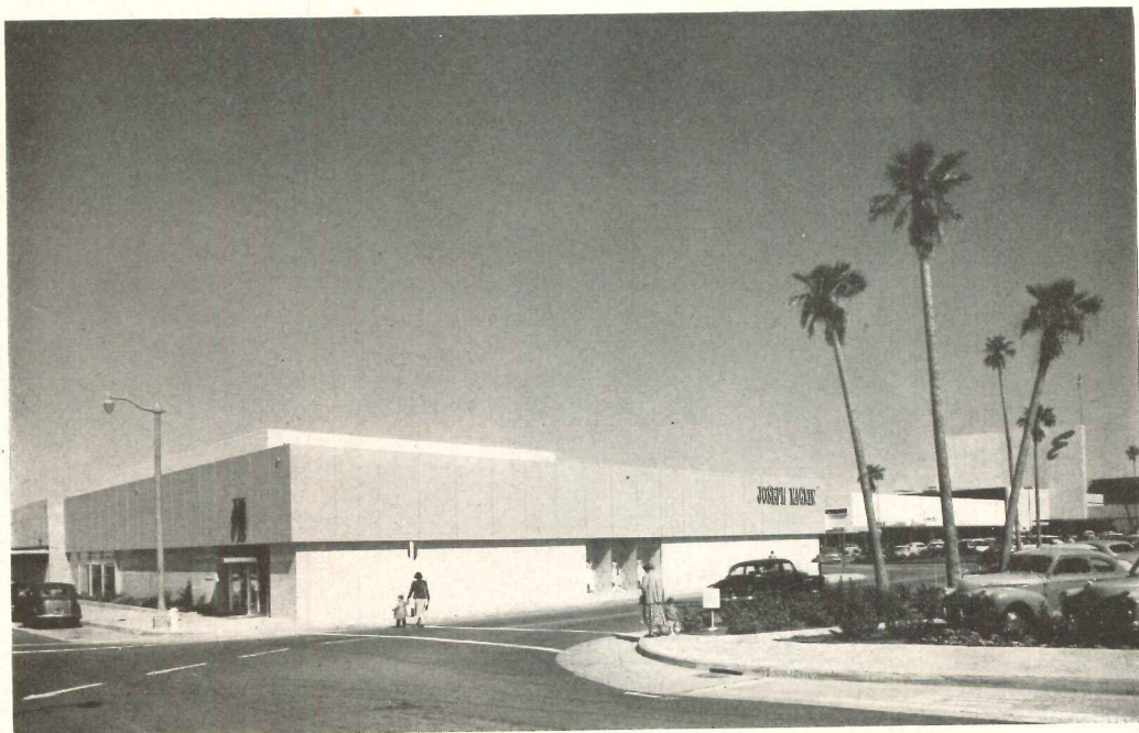
Lower walls are of Travertine marble; upper walls in painted concrete with wide grooves delineating a modular pattern
