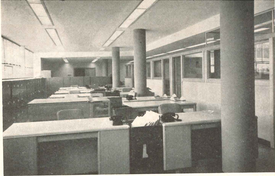
Interior trim is white birch, floors are asphalt tile, ceilings acoustical plaster. Overhead fluorescent lighting was designed to eliminate shadows, need for desk lamps
