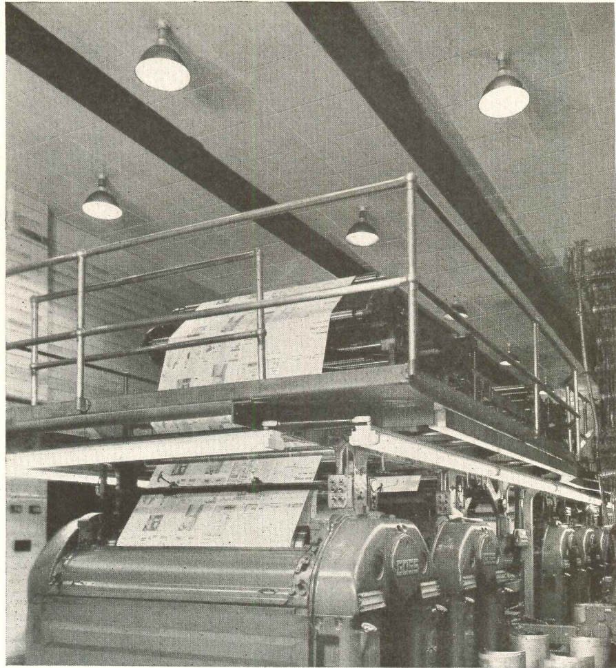
Grease and ink spray present no cleaning problem in this press-room. The fire-safe acoustical ceiling of Perforated Asbestos Board can be readily washed or repainted whenever necessary.
