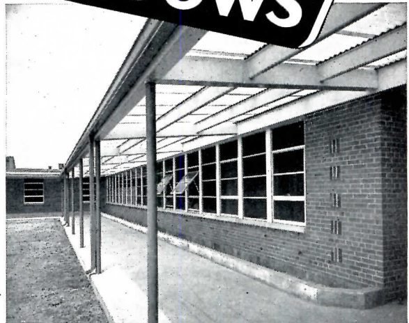
Northeast Jr. High School, Kalamazoo, Mich. Louis C. Kingscott — Architect Miller Davis Co. — Contractor
