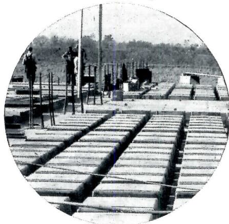
Two-way waffle design using Ceko-Meyer Steelforms permits longer spans, resulting in larger uninterrupted floor areas.
