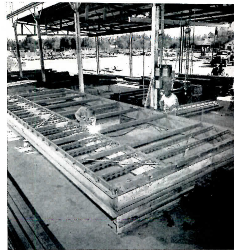
Steel frames are welded at shop
