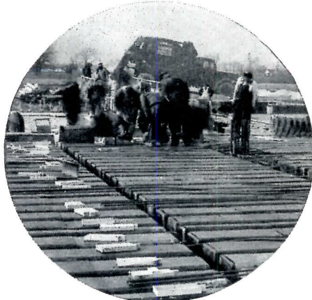
One-way Ceko-Meyer Steelforms also save steel and concrete, thus reducing dead load.
