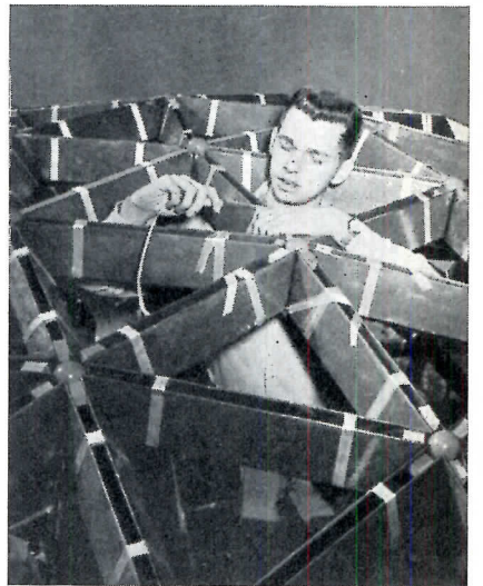
Tulane student taping cardboard triangles for added strength
