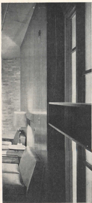
Plaster was virtually eliminated; concrete ceilings (bottom of nine-inch floor slab) were rubbed and given one coat of rubber latex paint; cinder block walls got two coats; some walls glazed brick
