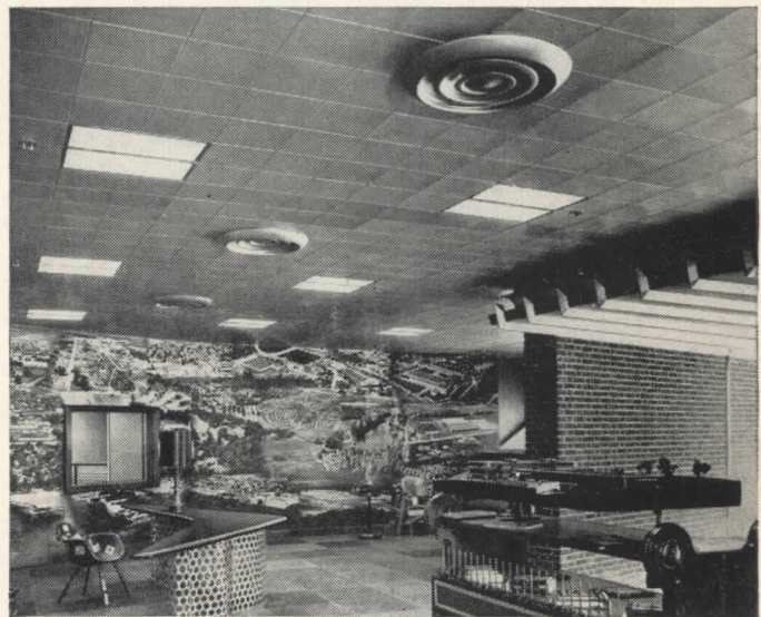
Discarded machine parts from Springs' own plants have been used to make most of the furniture throughout the offices. In the main lobby, the sound-absorbing ceiling of Arrestone with a bare mill finish blends with the metal furniture and fixtures.
