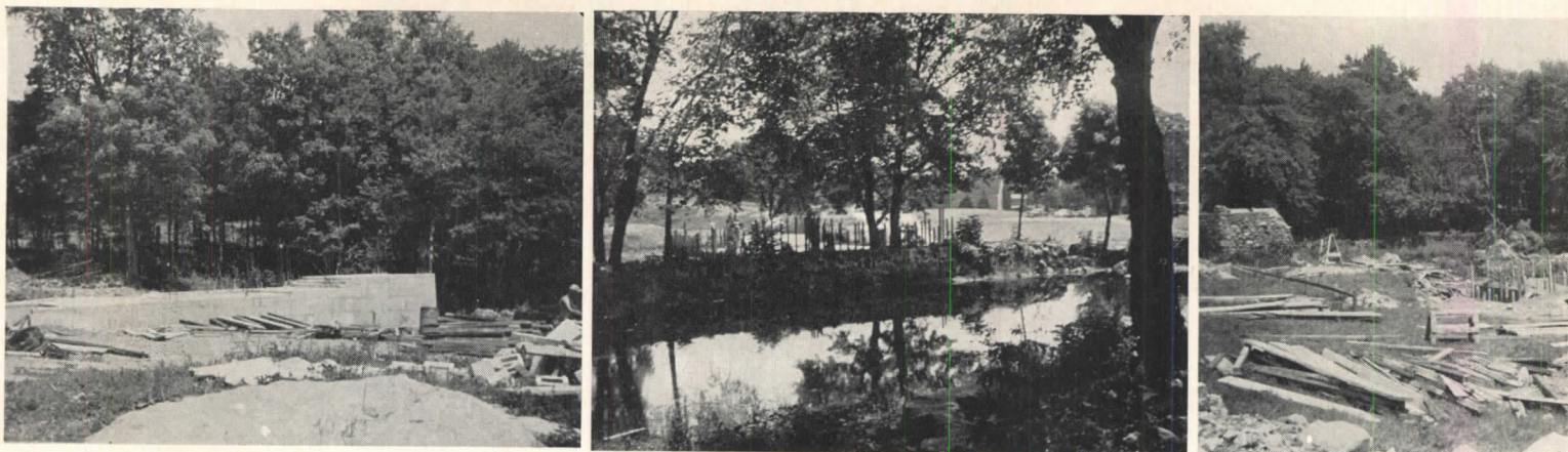
Three Chapels under construction: the pool glimpsed in center photograph is central in site plan (opposite)
