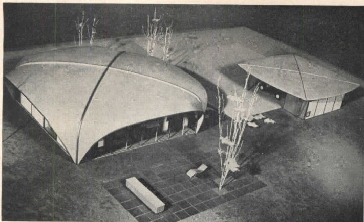
Plastic "House of 1964" designed by architect Eliot Noyes for General Electric — so far only a model for touring exhibits — has stressed-skin roof of two bonded plastic sheets, supported by aluminum ribs. Walls, partitions and floors are also of plastic. Lowered ceilings over bedrooms are made of a translucent plastic containing luminescent pigment which is electrically lighted. Circle in living room revolves
