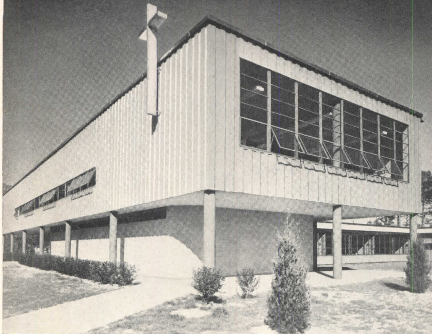
Notre Dame School, Biloxi, Miss. Wm. R. Allen, Architect Joseph Molitor, Photographer
