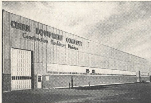
Clark Equipment Company, Construction Machinery Division, Benton Harbor, Mich., 45,630 sq. ft. of 2" Tectum plank for wall insulation.
