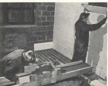
"Foamed polystyrene . . . has been used as an insulating back-up for concrete block walls, where it also formed the plaster base, thus eliminating furring, lath and vapor barrier."
