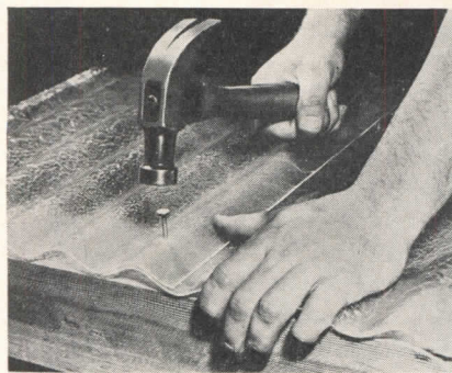
"The structural function (of corrugated reinforced plastic sheets) is combined with enclosure and light transmission, often simultaneously meeting a shatter hazard as in industrial buildings."
