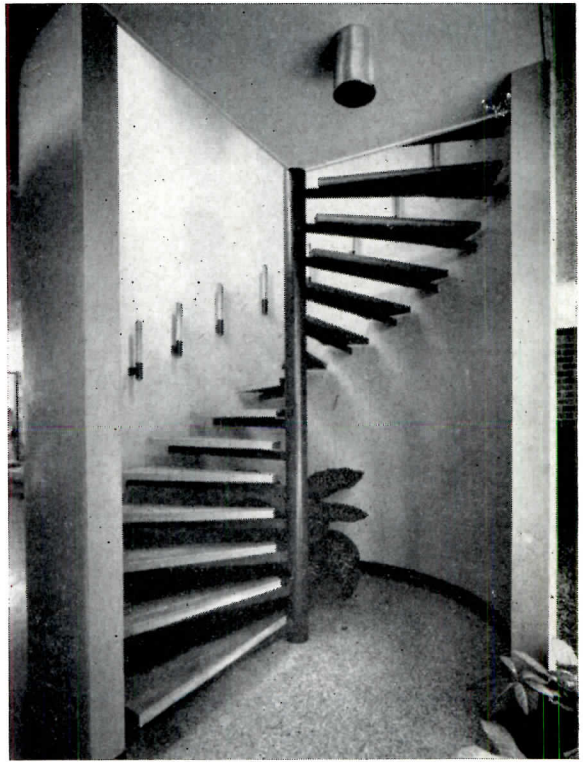
Viewed from below, the Tiller staircase (see also photo above) displays an open lightness of treads. Vertical grips replace handrail and form a decorative pattern. (Plan, page 114.)
