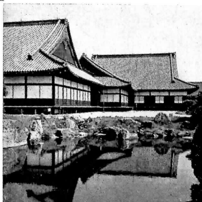
Left, Tana, a recess with wooden shelves. Below, the main buildings, Nijo Palace, graduated in harmony with the garden
