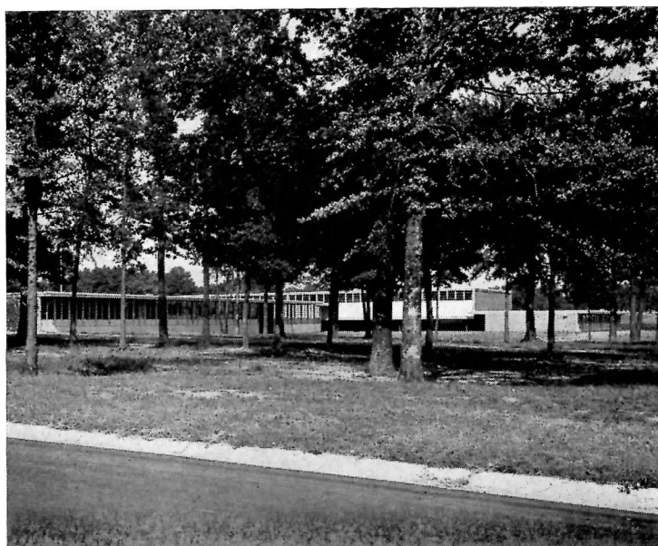
Courtyards and existing trees are invaluable assets
