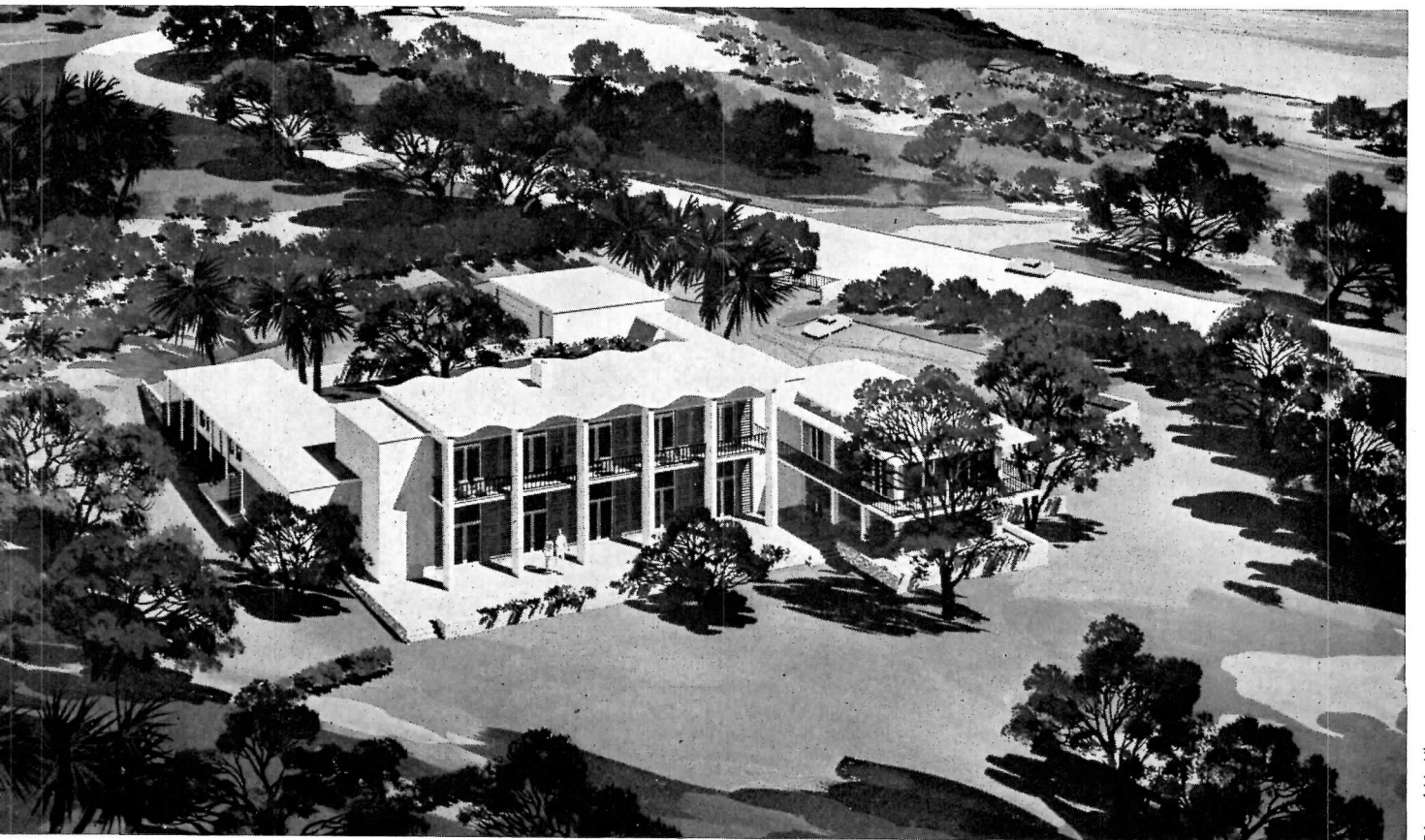
DAKAR, FRENCH WEST AFRICA; Consul General's Residence; Moore & Hutchins, Architects. Designed for a tropical climate, the building makes features of protection devices. Balconies and roof overhangs permit the large windows to be open during rainstorms
