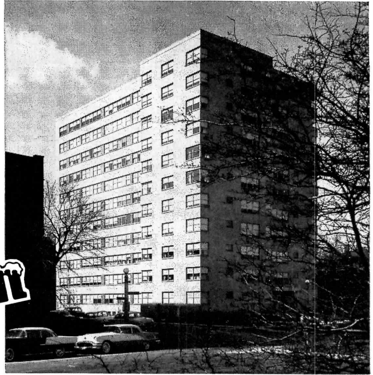
4200 Marine Drive Apartments, Chicago, Ill. Architect: Lewis Simon. Mech. Eng.: Arthur Wallace. Installing Contractors: Midwest Eng. & Equipment Co., Economy Plumbing & Heating Co.
