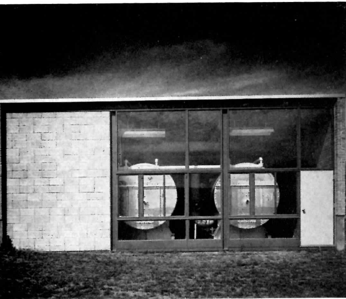
Boiler house is located at west end of campus
