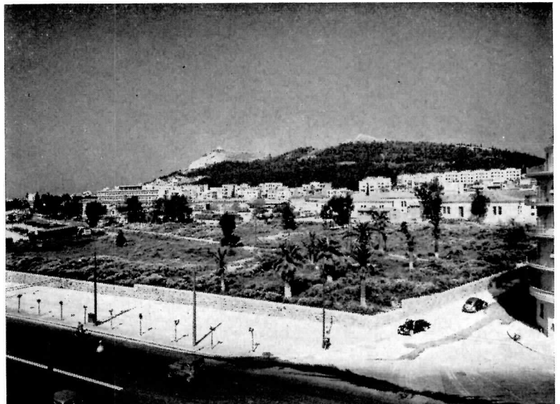
The sloping site on Queen Sophie Avenue
