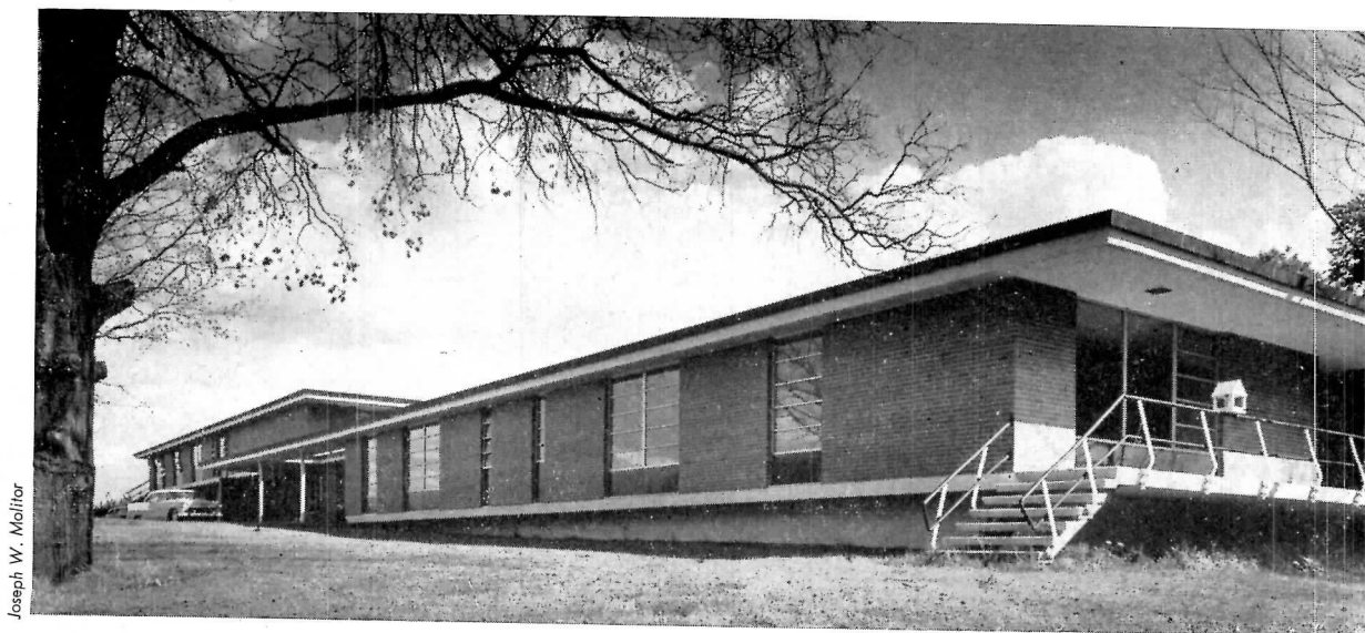
The large playroom is the scene of much of the training effort, since the three-year-old must not be pushed too hard. The regular classrooms are three separate units in a finger-plan scheme, as a wing extending out from the residential building. Costs of the reinforced concrete buildings was $11 a square foot, or a total of $300,000
