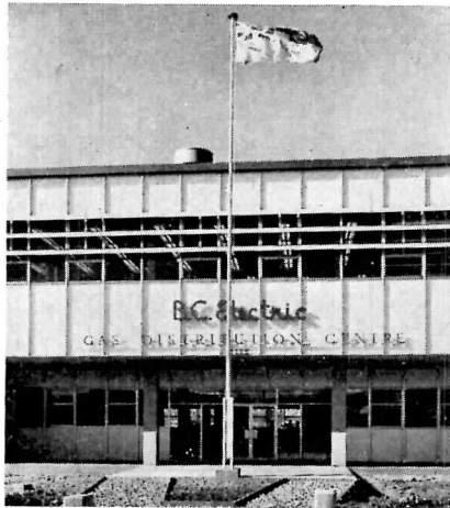
Service headquarters for B.C. Electric's natural gas distribution system, Burnaby; design by B. C. Electric Engineer Company
