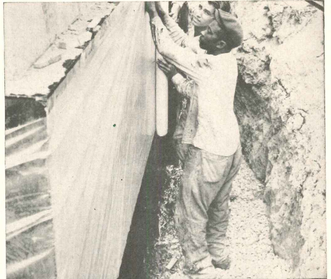
ON OUTSIDE OF FOUNDATION—mop with tar, apply VISQUEEN film, backfill and say goodbye to moisture ills for life of building.
