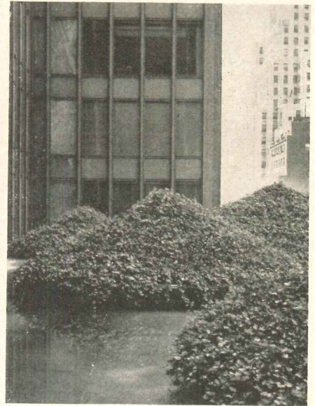
Finished garden on a fifth-floor terrace of Seagram Building gives a pleasant down-view from windows above
