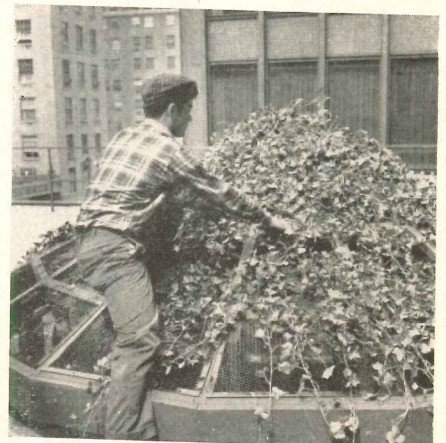
Workman spreading ivy runners out conically between planting boxes to give an immediate finished effect. Next, ivy was attached to wire mesh to prevent it from being blown out of position
