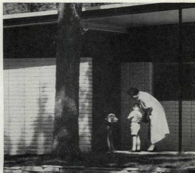
Design interest is achieved with coarse-textured block laid in a stacked bond
