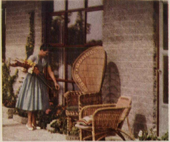
Living concrete in integrally colored 4"-high split block
