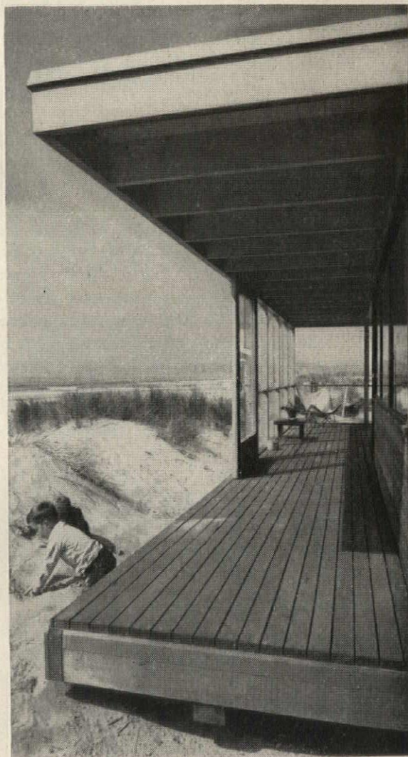
How to have your beach house on the sand, but not in it — set the house on wood piles several feet above the dunes, provide generous walkways of separated wood strips to filter out tracked-in sand. Note generous frame overhang, vital for sun protection. Francis J. McCarthy, architect.
