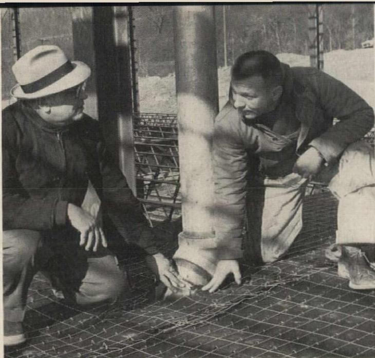
Snug fit of Steeltex around drain pipe at Canevin High School is shown by Joseph V. Cutuly, job superintendent (l.), and Foreman Dean Regan. Mr. Cutuly says, "Steeltex takes more punishment during installation than a sheet material, goes down faster and is much easier to handle."
