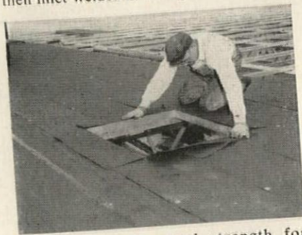
Tectum has structural strength for through-opening cuts between spans. It is easily sawed or drilled on the job with ordinary wood working tools.
