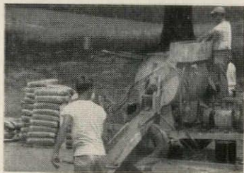
How it's made: For positive density control, BETOCEL is mechanically mixed in high speed machines. The wet mix flows easily into forms.
