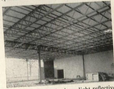
The finished deck is clean, light reflective and maintenance free. Tectum insulates, absorbs sound, is structural and noncombustible in accordance with Federal Spec. SS-A-118b.
