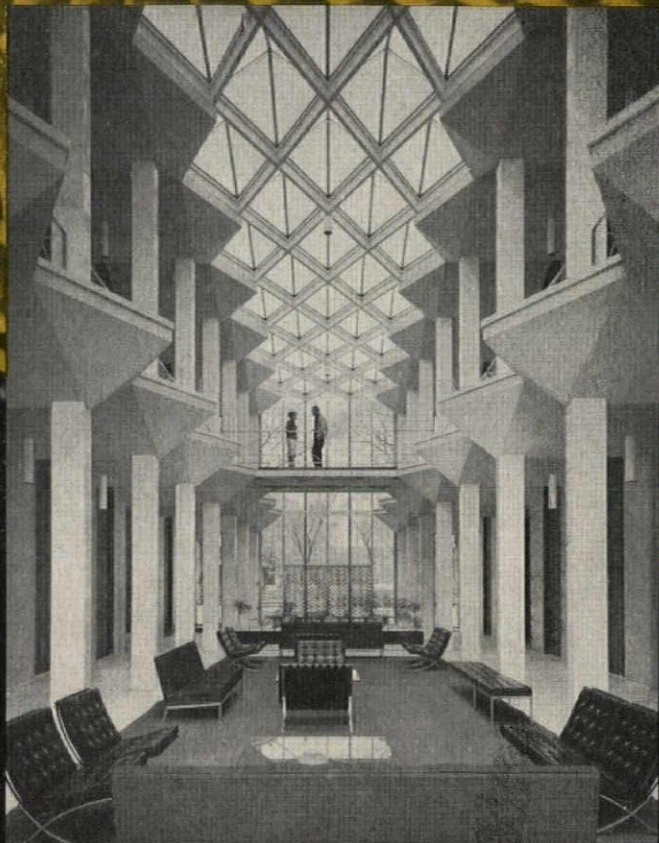
Concrete structural members in the McGregor Memorial Conference Building, Wayne University, Detroit, are beautified with plaster. A base coat of RED TOP* Cement Plaster on USG® Diamond Mesh Metal Lath is finished to a dense, durable surface with RED TOP* Gauging Plaster and Lime. Architect: Minoru Yamasaki & Associates, Birmingham, Mich. Plastering Contractor: M. A. Santoro, Inc., Detroit, Mich.
