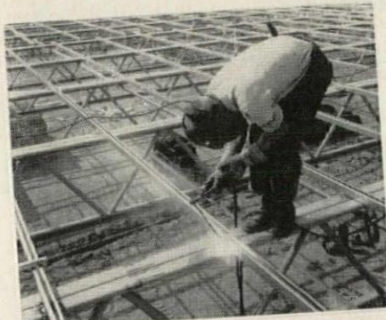
Welding at each joist crossing provides lateral strength and continuous beam action. Note weld is hidden from view below, by joist — no painting required.
