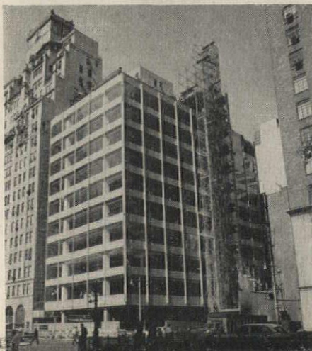
An early-August progress photo of World Headquarters for the Pepsi-Cola Company on New York's Park Avenue. The 11-story, 126,000-sq-ft structure is due to be occupied about the end of next month. Skidmore, Owings & Merrill, architects; Severud-Elstad-Krueger-Associates, structural engineers; Slocum & Fuller, mechanical and electrical engineers; George A. Fuller Co., general contractor
