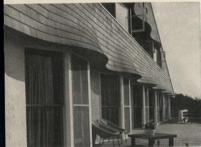
Architects George Nelson and Gordon Chadwick answer a tough design problem — providing interesting weather protection to beach home where all rooms have windows facing seaward. Answer: a fresh design motif suggestive of rolling surf — undulating "eyebrows" of weathered silver-gray wood shingles. Ezra Stoller, photographer.
