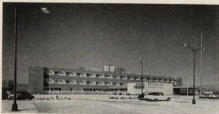
MCDONOUGH HOSPITAL, MACOMB, ILL. TROY-PLANNED LAUNDRY FOR ARCHITECT LANKTON-ZIEGELE-TERRY AND ASSOCIATES, PEORIA, ILL.
