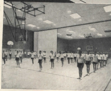
Shadle Park High School, Spokane, Washington, Culler, Gale, Martell and Norrie, Architects
