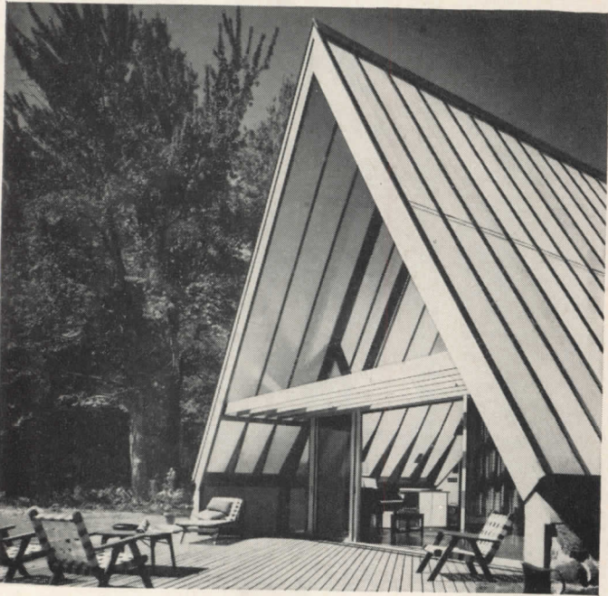
Using bolted A-frame members for rigidity and strength, ceiling and walls of this home combine to provide internal spaciousness while creating an unusual peak effect. Architect: Thomas C. Babbitt.
