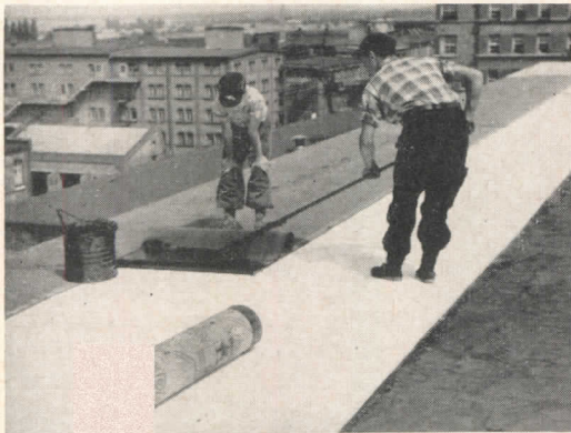
Figure 5. On flat roofs, insulating polystyrene foam sheets are laid on top of a layer of hot asphalt applied over a dry asphalt emulsion
