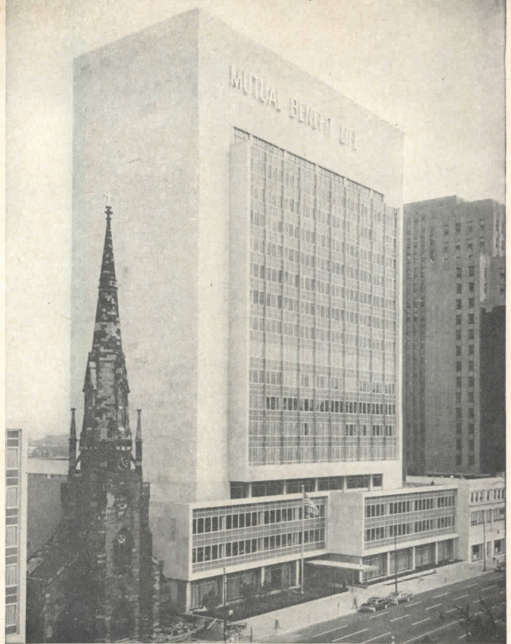
The Mutual Benefit Life Insurance Building, Newark, N. J., is one of the city's most modern landmarks. (Architects, Eggers & Higgins, New York City; Design Engineers, Syska & Hennessy, New York City; Fixture Manufacturer, Gruber Lighting Inc., Brooklyn, N. Y.; Installation, The Beach Electrical Company, East Orange, N. J.)
