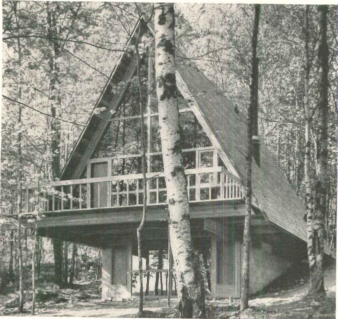
Tent-shaped A-frame vacation houses are equally at home on a coastline or in a woodland. Wood's easy portability adds to its economies. Architect: Richard Whiteman of Jyring & Whiteman.
