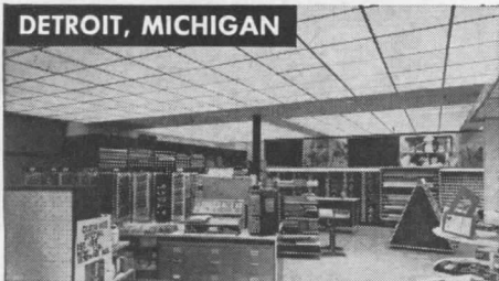
Circlgrid Luminous Ceiling installed in retail store
