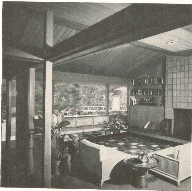
Exposed laminated beams and post supports, in concert with a plank ceiling and paneled bookcase-wall, set the tone for comfort in this modern living room; uphold wood's accord with other materials.
