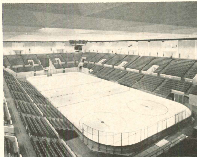
Tulsa Assembly Center is designed for multi-purpose use. The 55,000-square-foot area, which can be converted for ice hockey, can seat 6,500 on permanent seats, another 3,500 on the 24,000-square-foot floor. Steel trusses spanning 240 feet eliminate columns—there's not a bad seat in the house. To the left of the entrance (dark panels in facade) is a 100 foot
