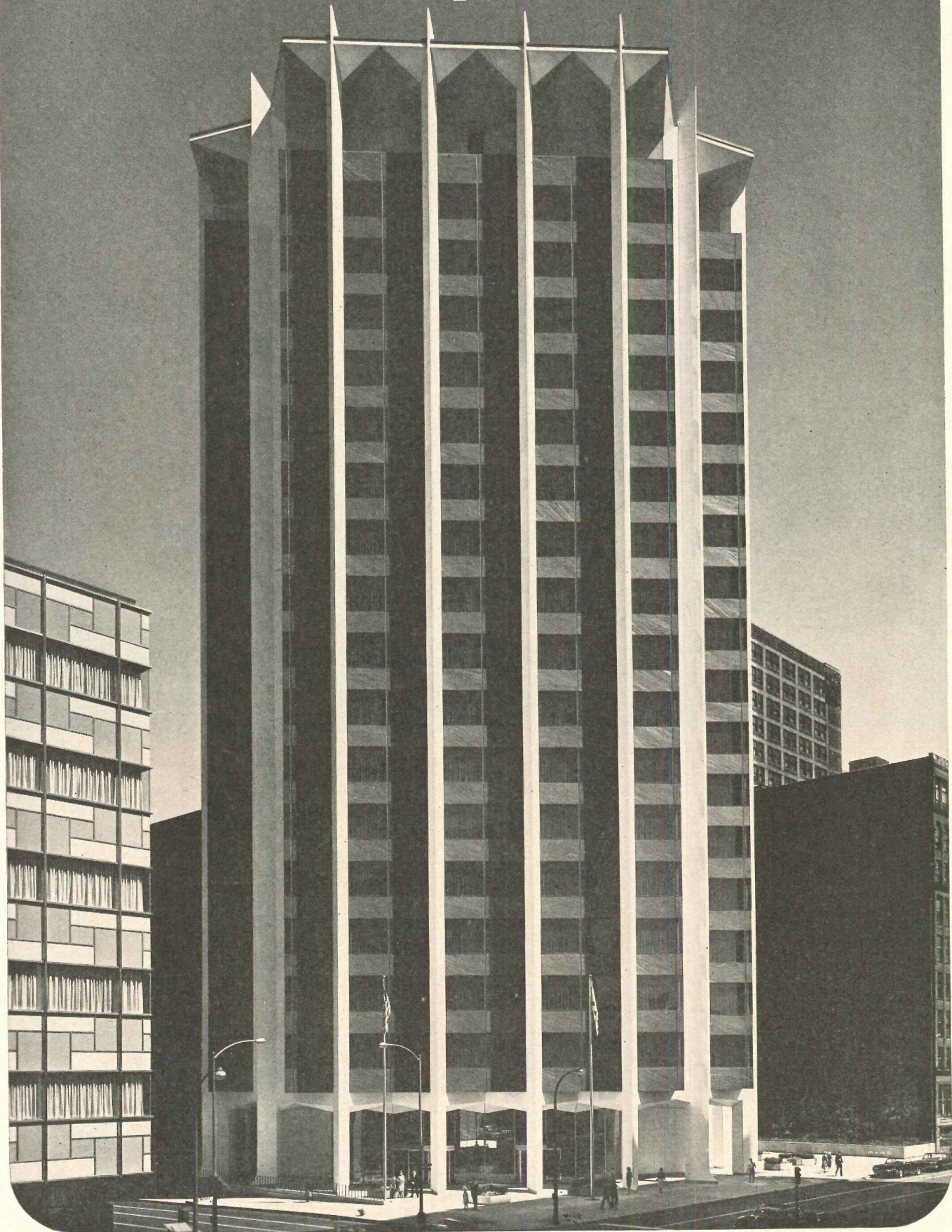
United States Gypsum Building, Chicago, Ill. Architects: The Perkins & Will Partnership. Glazing Contractor: Hamilton Glass Co., Chicago.
