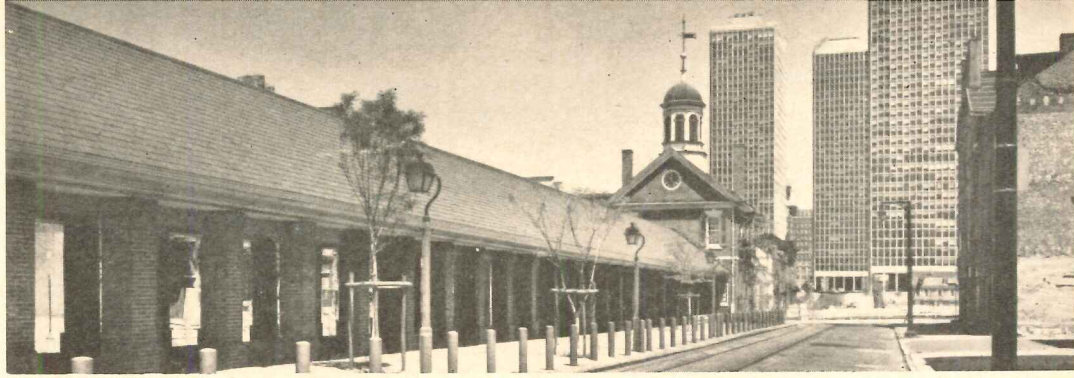
The towers in Society Hill designed by I. M. Pei were carefully sited to relate to certain historic structures designated for preservation. Headhouse, New Mar-
