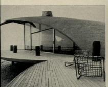
The interlocking frames put their back to the strong winds and send them harmlessly out to sea. The roof's glued-laminated Western Wood beams curve to the foundation where they are secured to treated wood pilings sunk in
