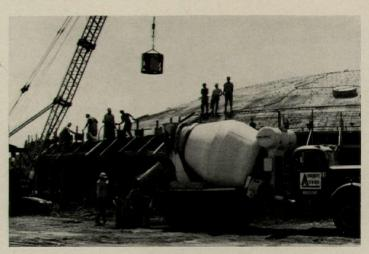
Concrete was placed over cement excelsior sheets which, in most areas, will be left exposed. Wherever possible crane and bucket were used for placement. In those areas which could not be reached by this method, concrete was placed by pump.
