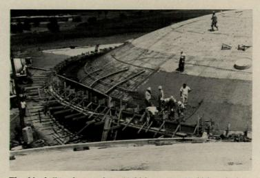
The thin-shell roofs range from 4" thick at top to 8" thick at the base and 16" thick at the tension ring. Domes are 33' high at center and 180' in diameter.
