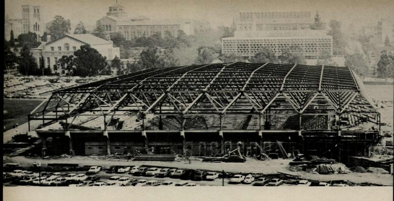
space frame. Panels are supported on the cantilever ends of the bents. Upper level concrete risers are exposed below the panels.
