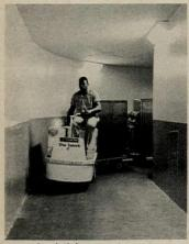
Special, fail-free train on ramp works 18-hour day of 90-minute round trips throughout hospital. Ramp for goods saves elevators for people, would speed evacuation in case of fire. Top-level truck delivery, below right, permits design of "upside-down" hospital.
