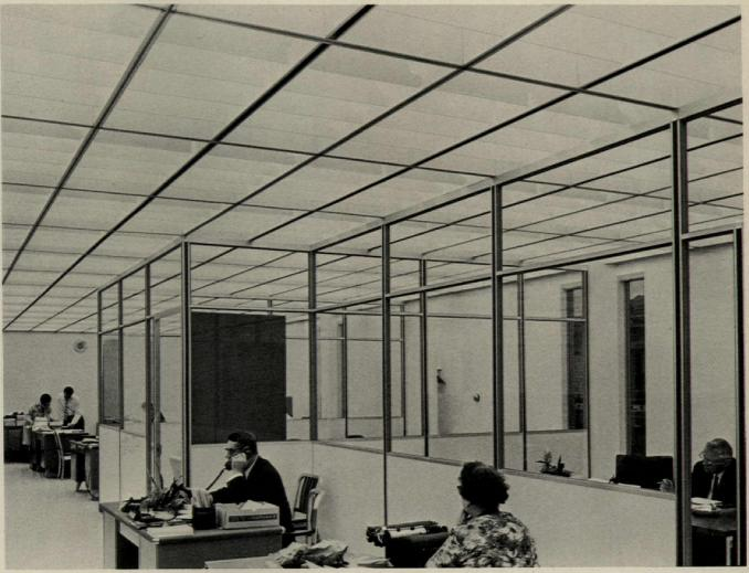
This is Quartette, the total integrated ceiling system. Lighting of 450 footcandles without glare. Complete air exchange. Unbelievable acoustics. And full partition support. All packed in custom-sized modules to fit your next job. There's no ceiling in the world to compare with it. Write for details. Be amazed.
