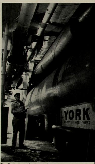
**Five York absorption type units,** with a total capacity of 3,312 tons, provide chilled water for the five buildings that make up the Lincoln Towers East group.
