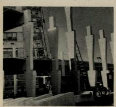
Standardized precast, prestressed concrete members were ready for rapid assembly the moment the foundation was
