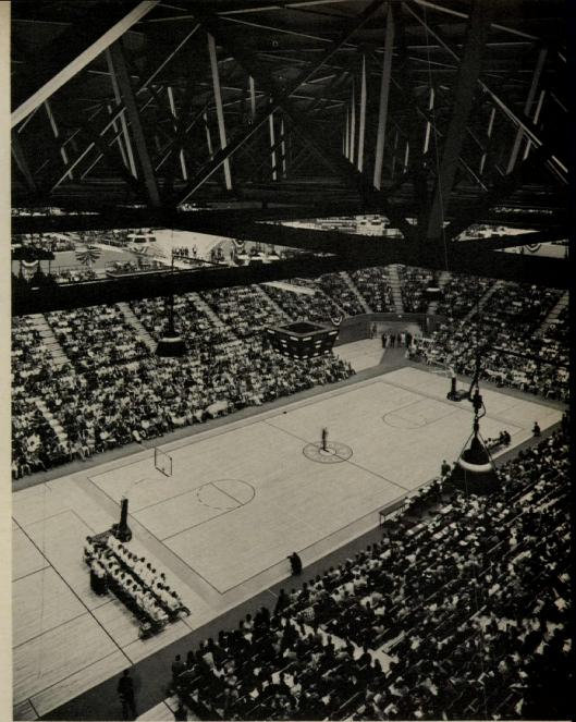
Economy resulted more from attention to ease of construction than to high theoretical refinement of structure. This largest horizontal steel space frame to date provided 120,000 square feet of clear space for the Pauley Pavilion at U.C.L.A.
