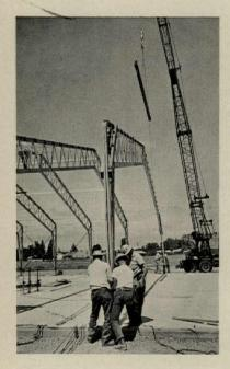
TRUS JOIST's perfect blend of wood and steel offers unique design freedom with economy. That blend provides much more too...light weight for easy erection and for savings in foundations, footings and bearing walls ... nailable top and bottom chords for the attachment of low cost roofing, ceiling and flooring materials... open webs for duct work and wiring... minimal deflection in spans up to 100 feet.
