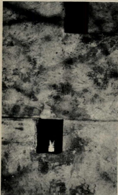
Two fountain details used in the Riis Park project: left, a horsetail jet concealed in a recess of a step, and right, a vortex suppressor to limit height of water supply for a series of concrete troughs.
